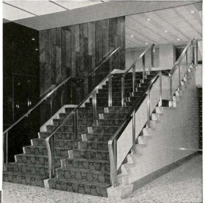
Handrails of the gracious main stairway in the Queen Elizabeth Hotel are fabricated from Anaconda Nickel Silver.
