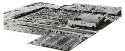
Lawrence Plaza - Toronto. Lawrence Plaza with its 38 shops including Morgan's Department Store is heated from a central Coal-fired Boiler room.
