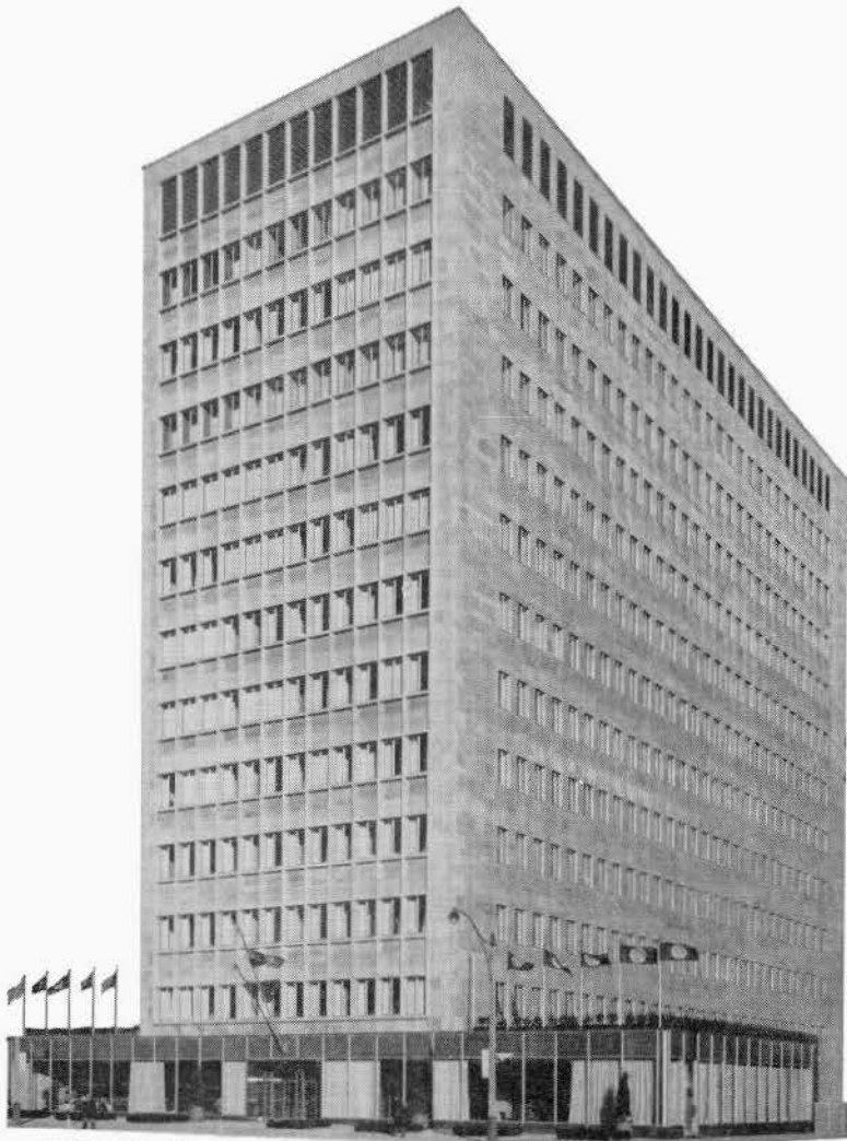
SHELL BUILDING 505 University Avenue, Toronto Architects: Marani and Morris Consulting (mechanical) Engineers: Wiggs, Walford, Frost and Lindsay General Contractors: Redfern Construction Company Limited Trane air conditioning equipment installed by: Steen Mechanical Contractors, Ltd.
