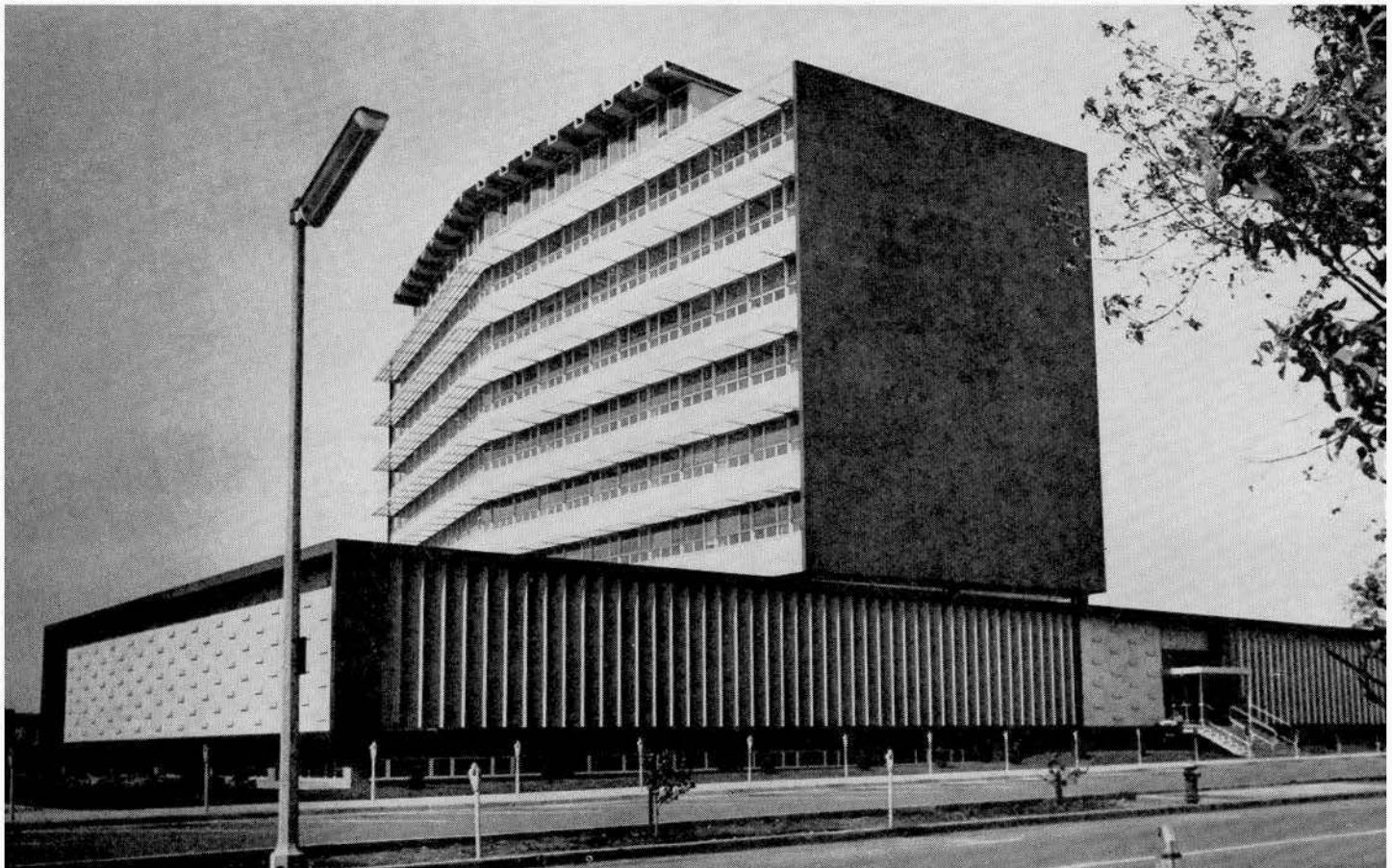
Louvered wall of the general office
