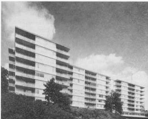
Structure: Benvenuto Apartments, Toronto, Ont. Architects: Page & Steele Cons. Structural Engineers: Hooper & Yolles General Contractor: L. S. Yolles
