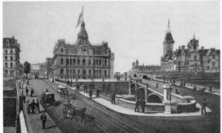
Post Office and Bridges
