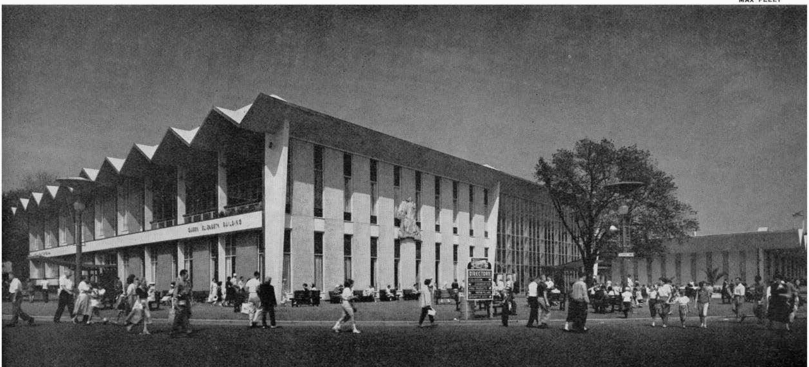
Overall view from south-west
