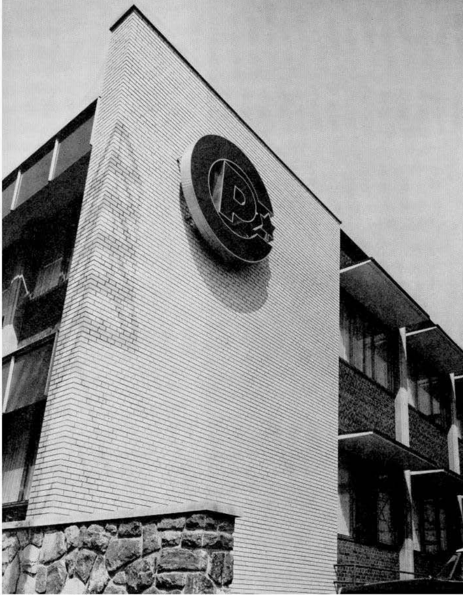
Detail of east elevation
