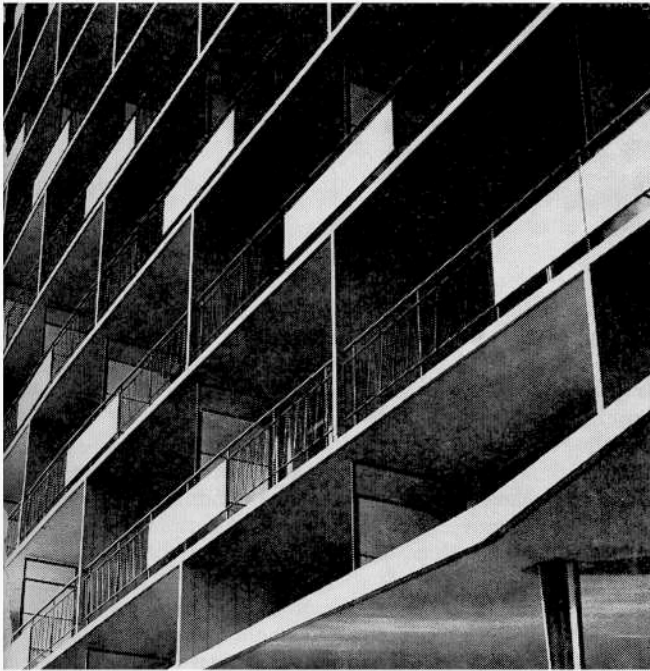
Detail of balconies
