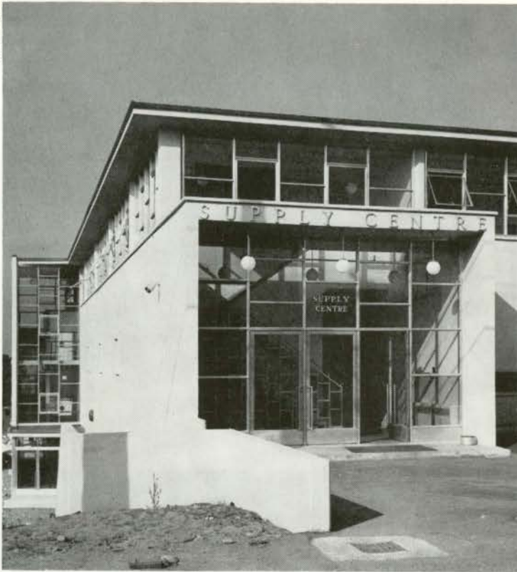
Supply Centre main entrance
