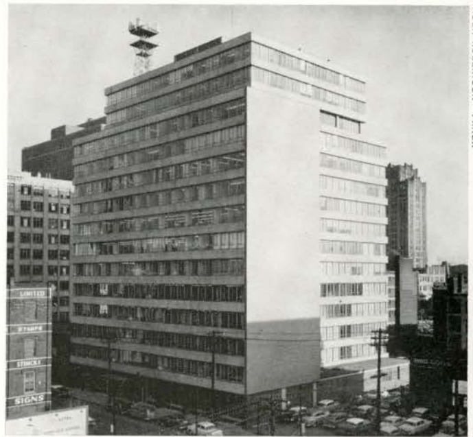
View from the north-west. The plain masonry wall is in green semi-glazed imported brick.
