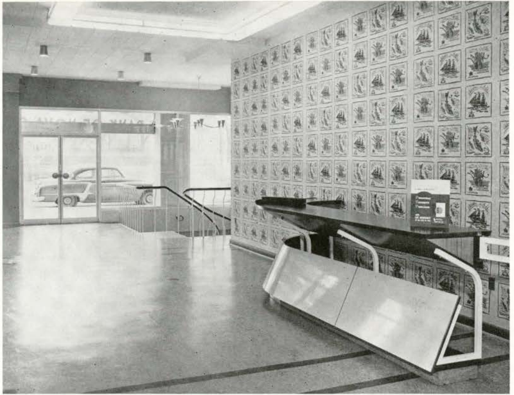
Interior looking toward entrance
