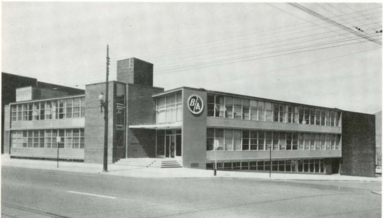
View from the south-east
