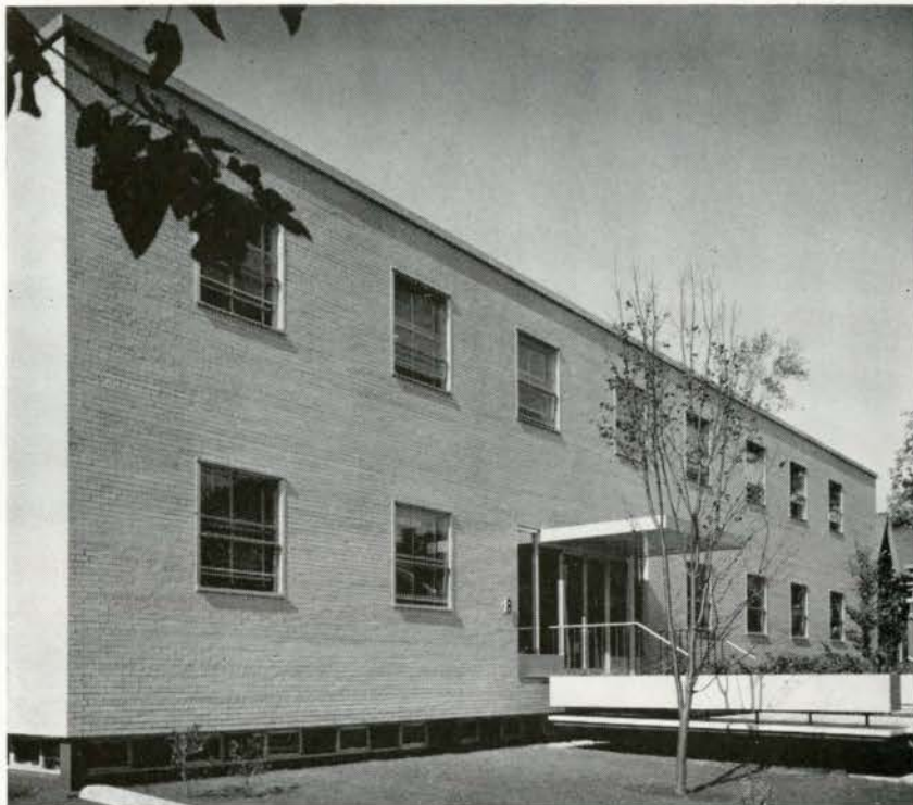
Main entrance front
