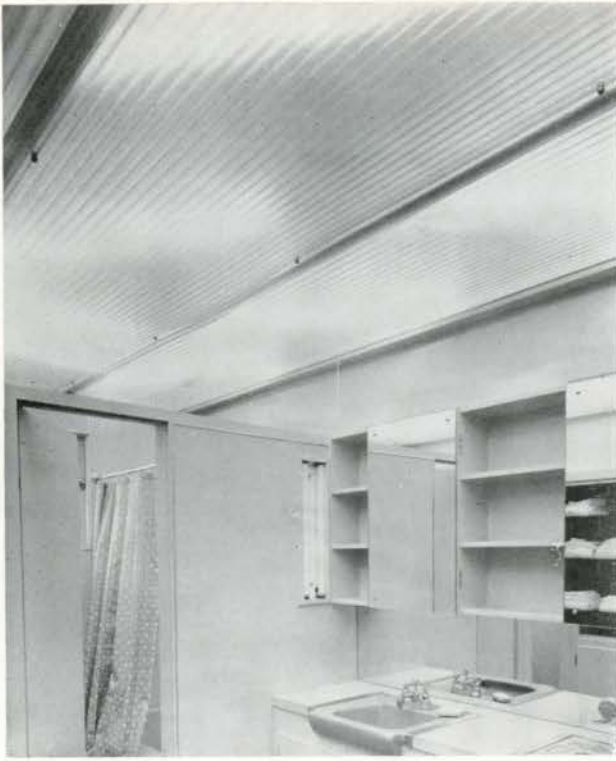
Bathroom with arborite walls and polyrein ceiling
