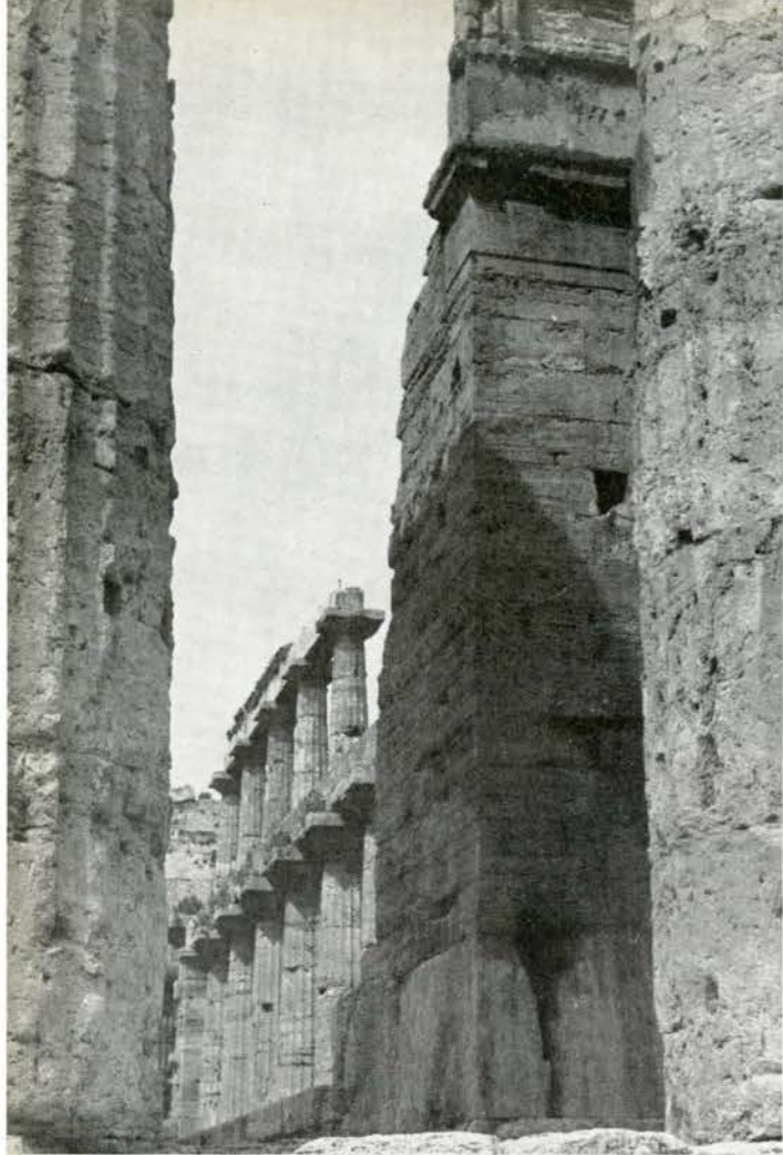
Paestum, Italy. Temple of Neptune; the interior was divided into three aisles by two rows of double-storied Doric columns.
