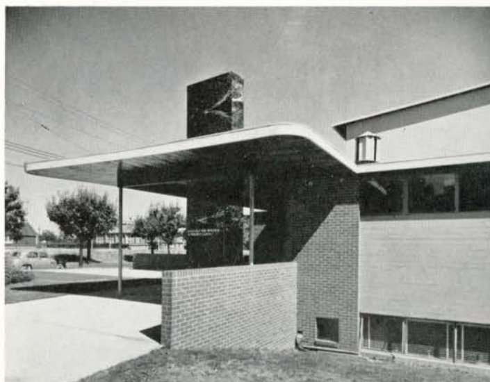
DETAIL OF ENTRANCE
