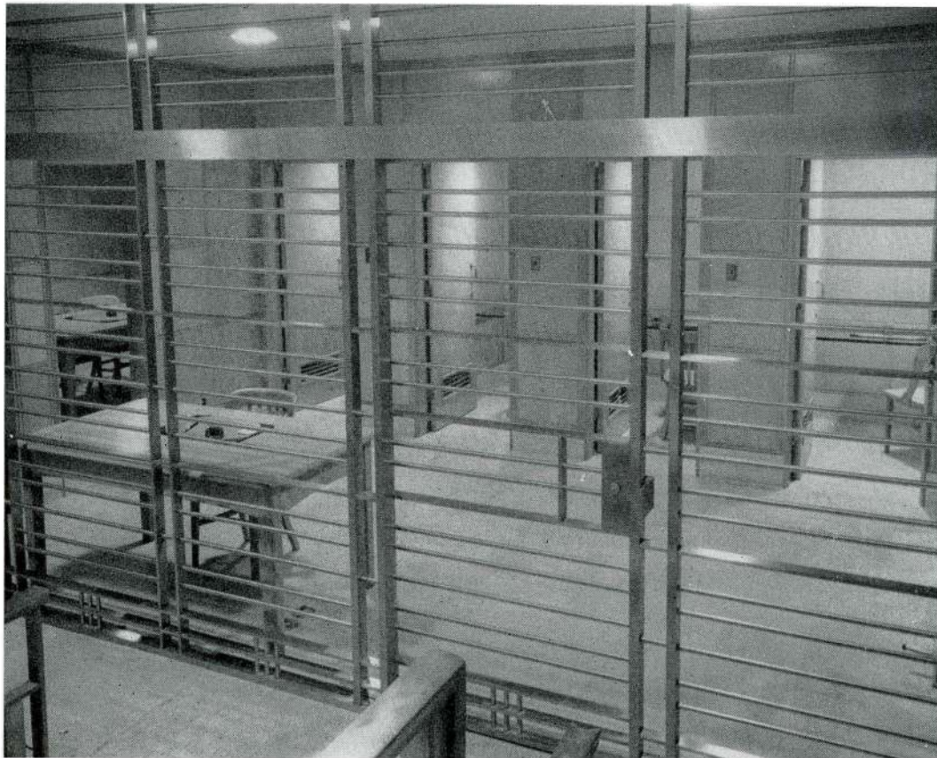
View showing Safety Deposit Grille and Coupon Booths.
