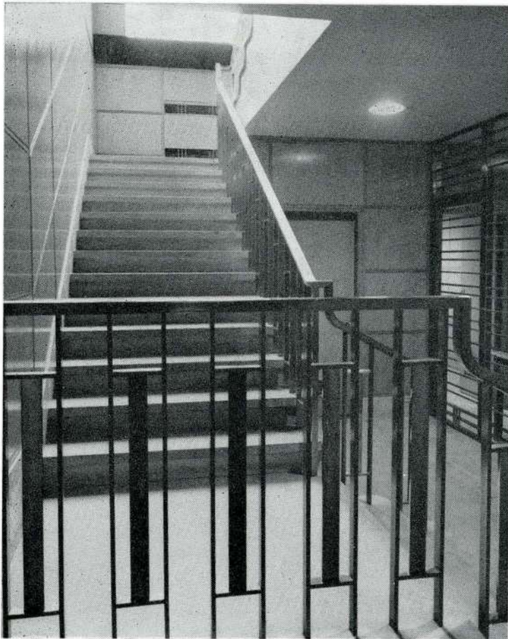
Detail of stair to Safety Deposit Department. Marble treads and risers. Stainless steel balustrade.
