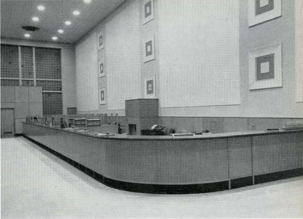
Counter and Book Lift. The Manager's Private Office is at the left of this view. All panelling is limed oak. The exhaust duct runs under the floor beneath the counter.
