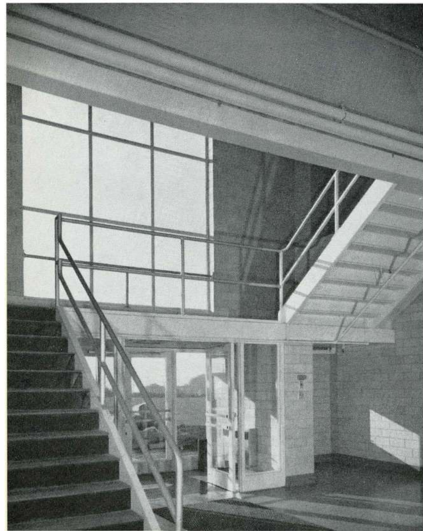
EMPLOYEES' ENTRANCE STAIRWAY
