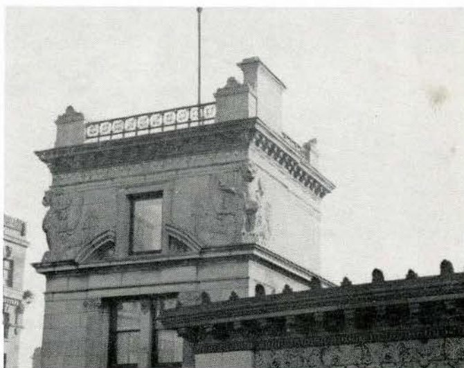
Cornice — Canadian National Railways Building, Montreal. Erected 1901.
