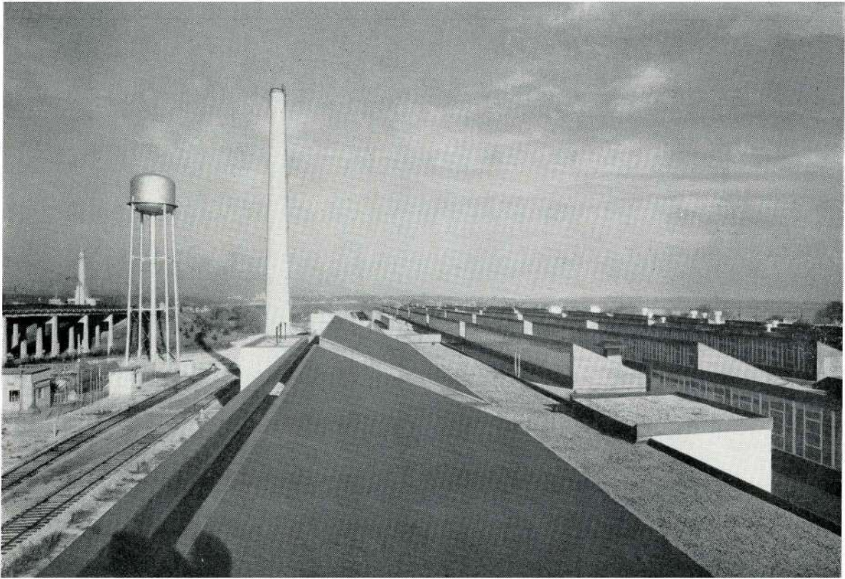
VIEW OF ROOF LOOKING EAST
