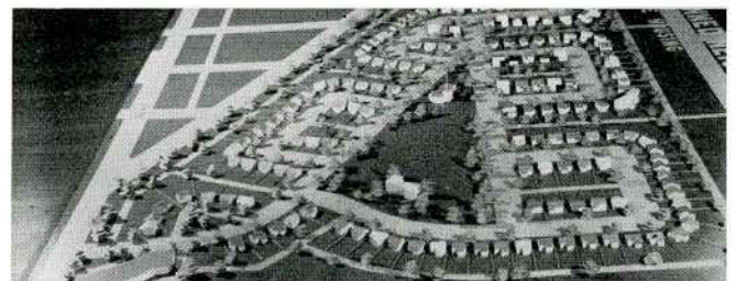
Wartime Housing Neighbourhood Development. (Under construction)
