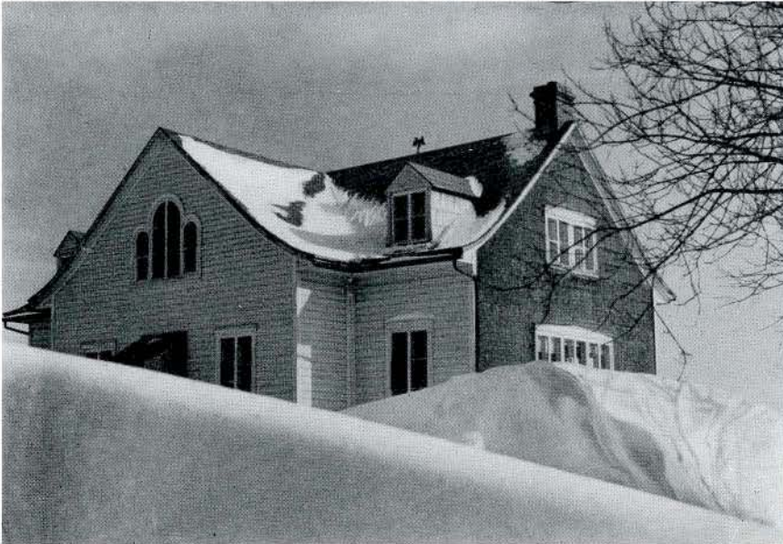
VIEW OF THE SCHOOLHOUSE IN WINTER
