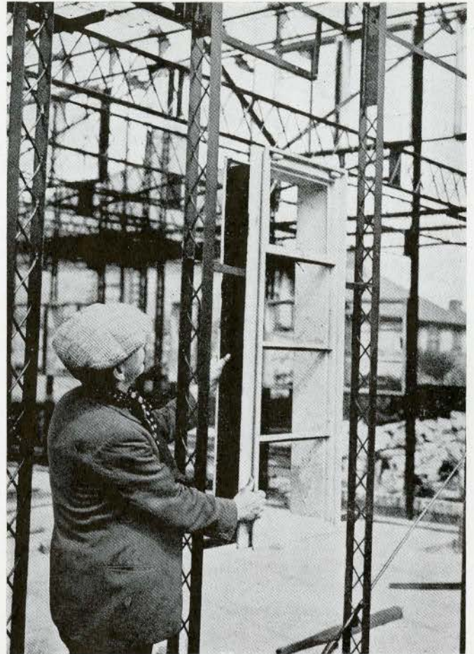
ERECTING WINDOW FRAMES IN UPPER FLOORS, BEFORE WALLS ARE ERECTED
