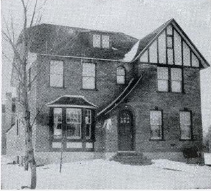
● COAL BLOWER—Quebec City, P.Q.
