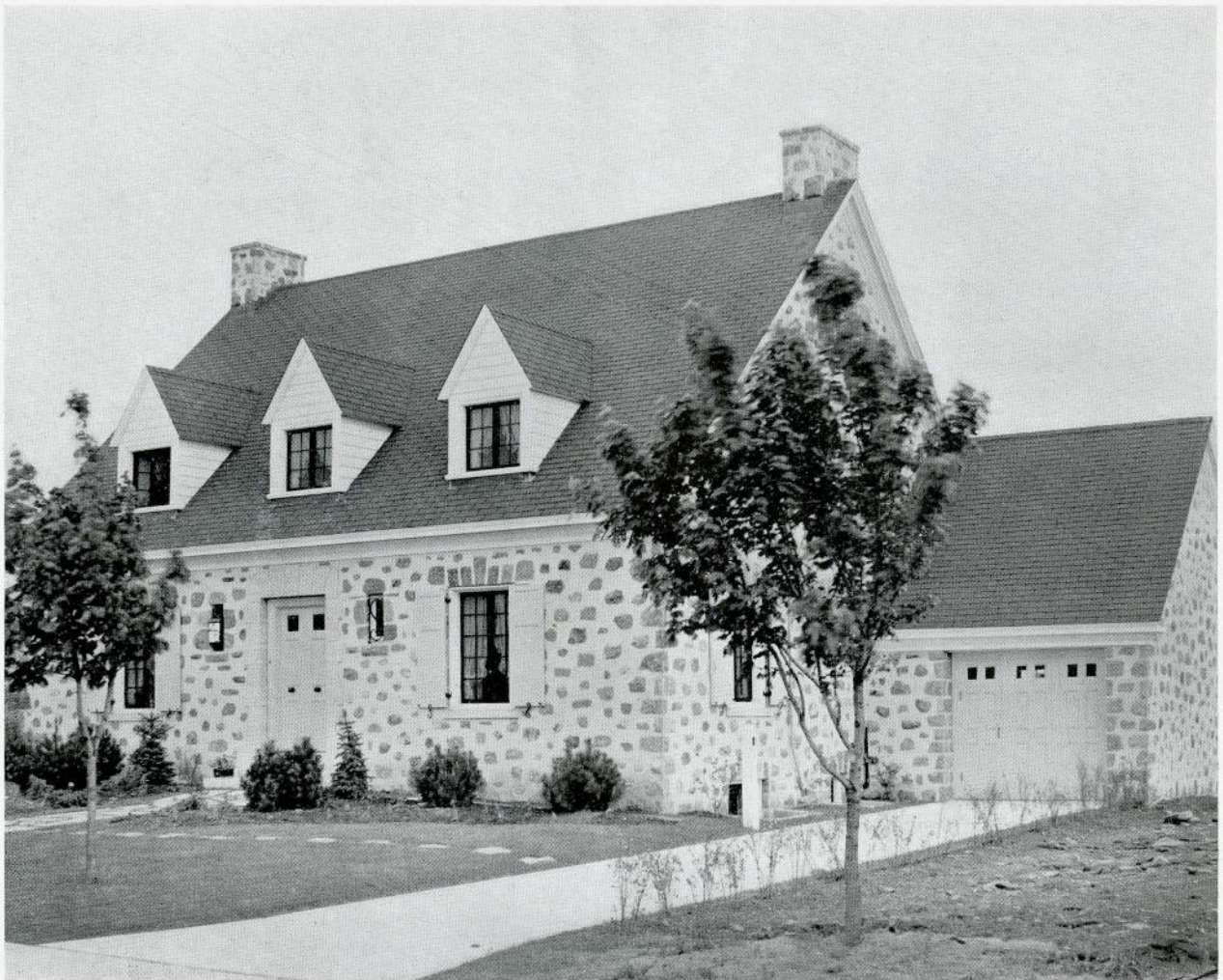
HOUSE OF MR. STANLEY STANGER, HAMPSTEAD, QUEBEC LAWSON AND LITTLE, ARCHITECTS
