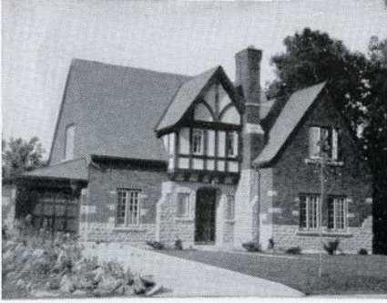
● OIL BURNER—Walkerton, Ont.
