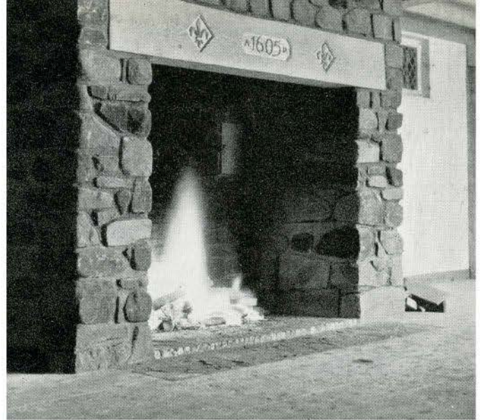
COMMUNITY ROOM AND GOVERNOR'S HOUSE FIREPLACES
