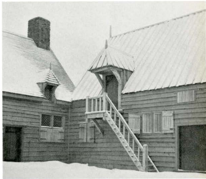
STOREHOUSE, LOOKING NORTH-EAST IN COURTYARD
