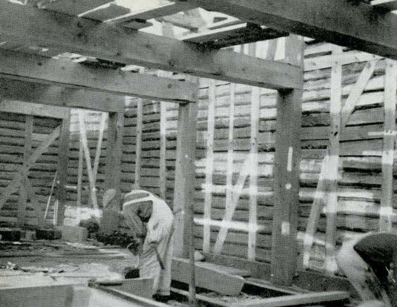
WALL CONSTRUCTION AND TIE BEAMS
