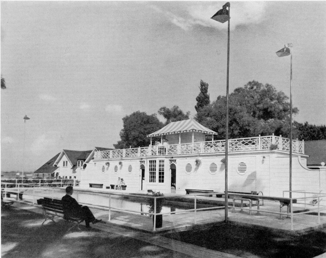
SWIMMING POOL AND BATH HOUSE, ROYAL CANADIAN YACHT CLUB, TORONTO MARANI, LAWSON AND MORRIS, ARCHITECTS
