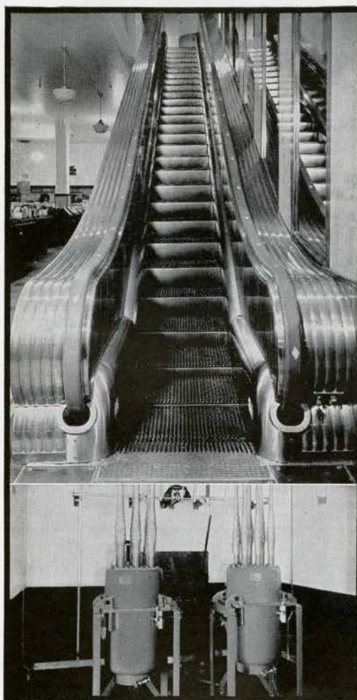
New F. W. Woolworth Store in Montreal, P.Q. Architects, F. W. Woolworth Engineering Staff in association with Archibald & Illsley, Montreal; General Contractor, Richard & E. J. Ryan; Electrical Contractor, Century Electric Co. Top view at left shows Westinghouse-Turnbull Electric Stairway of modern design. Lower view shows two Westinghouse Circuit Breakers which form part of the Electrical Substation in the basement.
