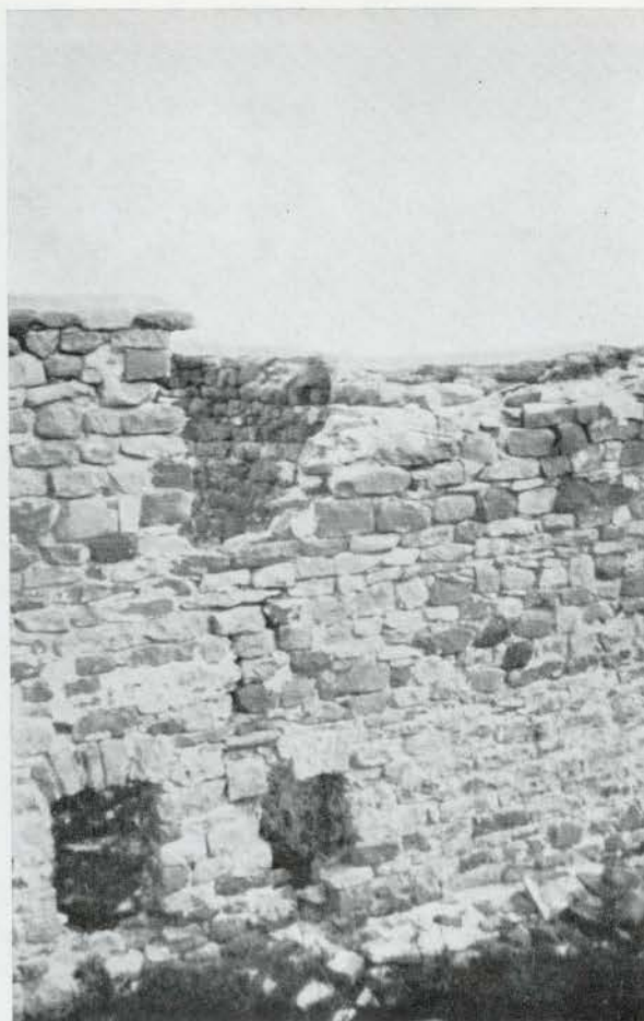
MASONRY WALL, FORT PRINCE OF WALES
