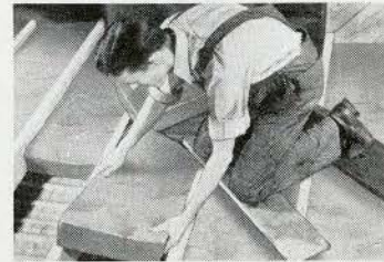
EASY TO INSTALL: Due to their semi-rigid construction, the new J-M Batts can be lifted, bent and applied in awkward places without damage. Application is speeded up.
