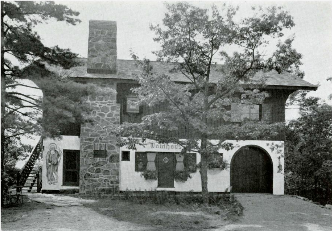
HOUSE OF MR. G. E. HACKNEY, SEIGNIORY CLUB LAWSON AND LITTLE, ARCHITECTS
