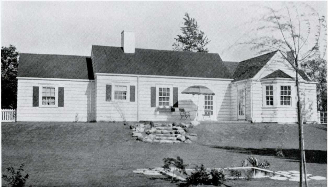
HOUSE OF MR. LEONARD D. DUECK, VANCOUVER WILLIAM FREDK. GARDINER, ARCHITECT
