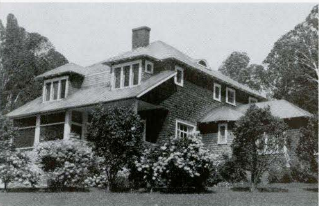
Residence of Mr. J. S. Norris, near Magog, Que., re-roofed with Anaconda Economy Copper Roofing by Douglas Bros., under the supervision of W. K. Gordon Lyman, M.R.A.I.C., Architect, Montreal.
