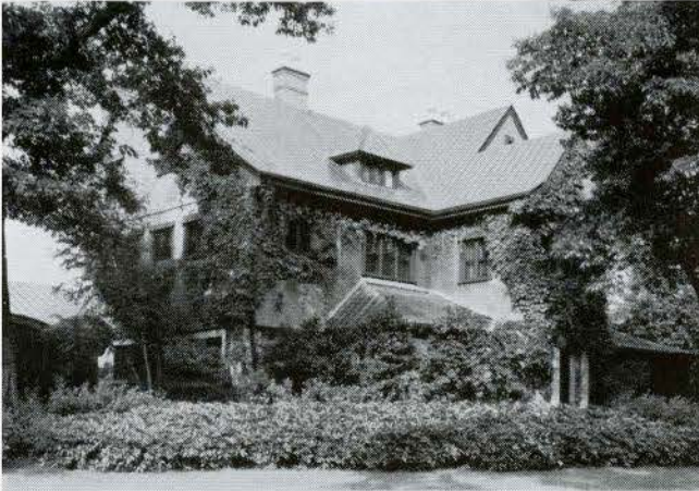
Residence of Mr. F. N. Southam, Westmount, Que., re-roofed with Anaconda Economy Copper Roofing by Douglas Bros., Montreal, supervised by Hugh Vallance, R.C.A., Montreal.
