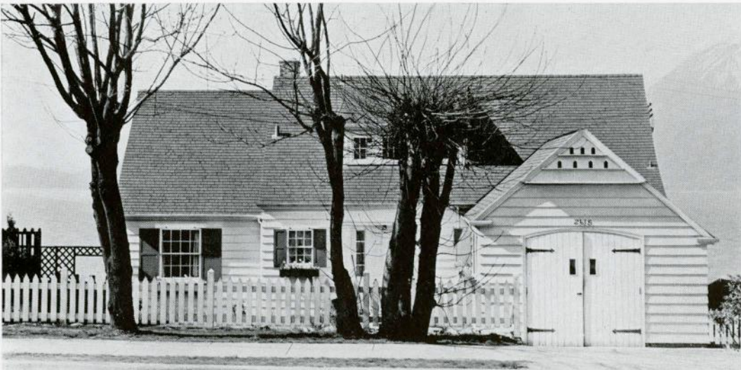
HOUSE OF MR. L. P. YOUNG, VANCOUVER C. B. K. VAN NORMAN, ARCHITECT
