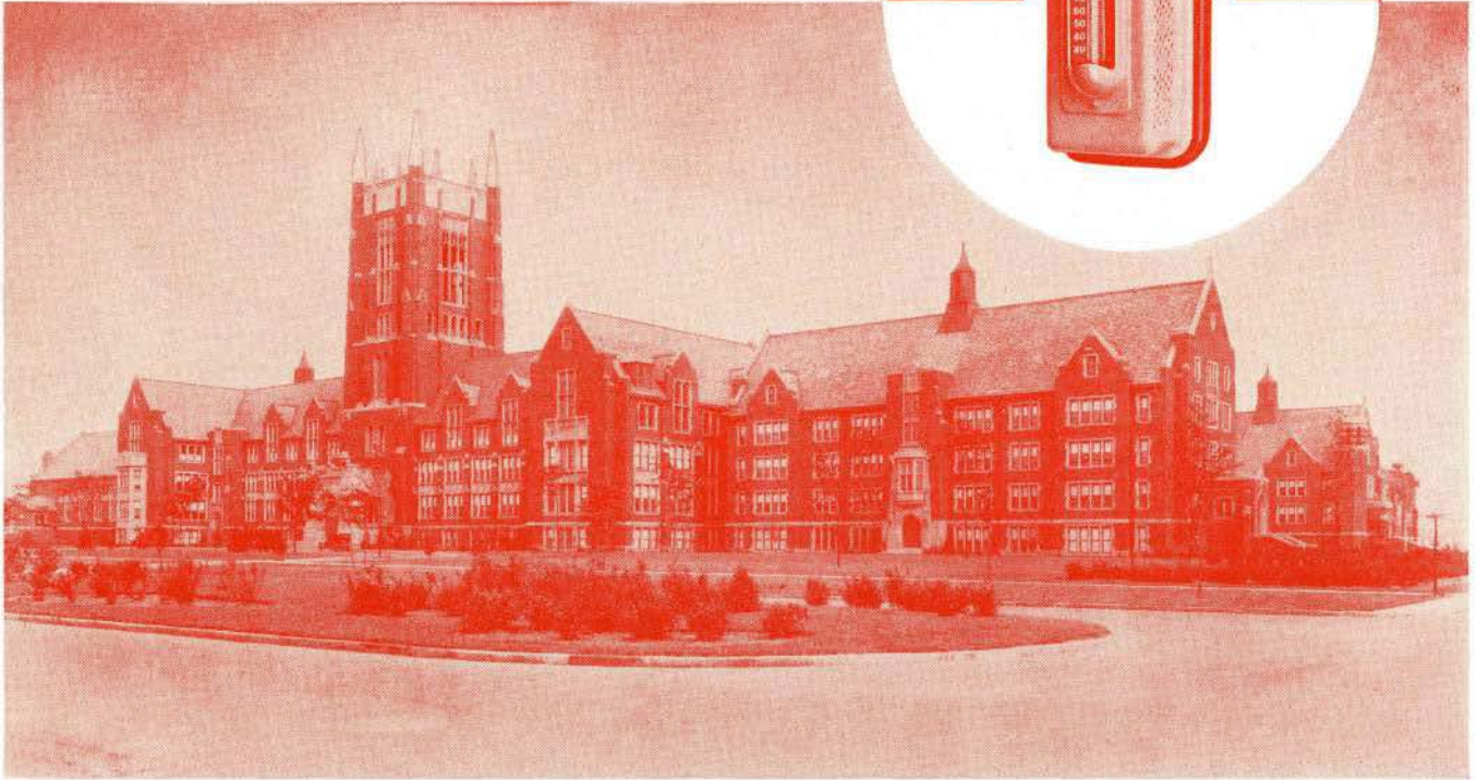
Sacred Heart Seminary, Detroit, Michigan. Architects: Donaldson & Meier. Mechanical Engineers: McColl, Snyder & McLean. Heating and Ventilating Contractors: Harrigan & Reid.
