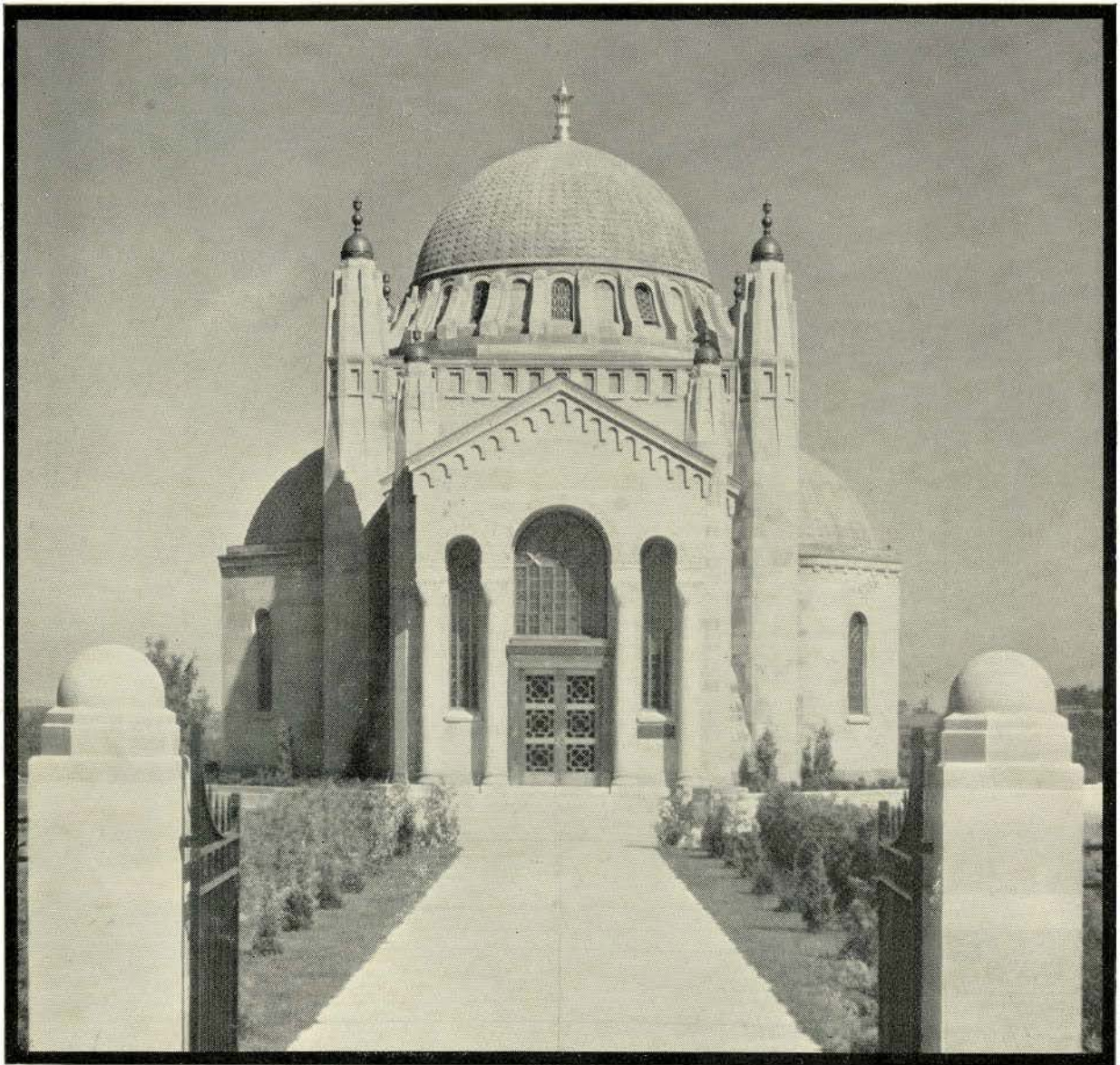
WEST ELEVATION, FROM THE ENTRANCE GATES
