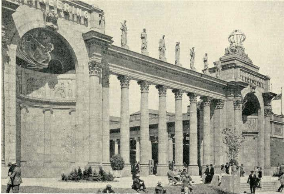
The pillared entrance to the Electrical and Engineering Building, Canadian National Exhibition, Toronto.
