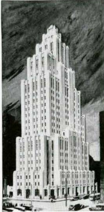
The Aldred Building, Montreal
