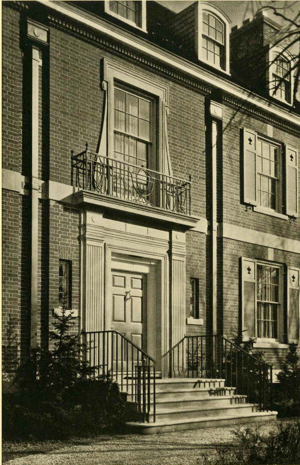
ENTRANCE DETAIL RESIDENCE OF H. C. WALKER, ESQ., TORONTO
