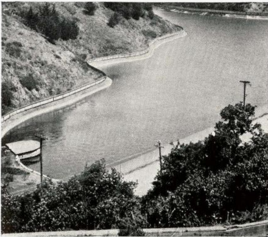
The water draining into this reservoir is only normally corrosive. A new reservoir, perhaps only 25 miles away, may supply water that is highly corrosive.
