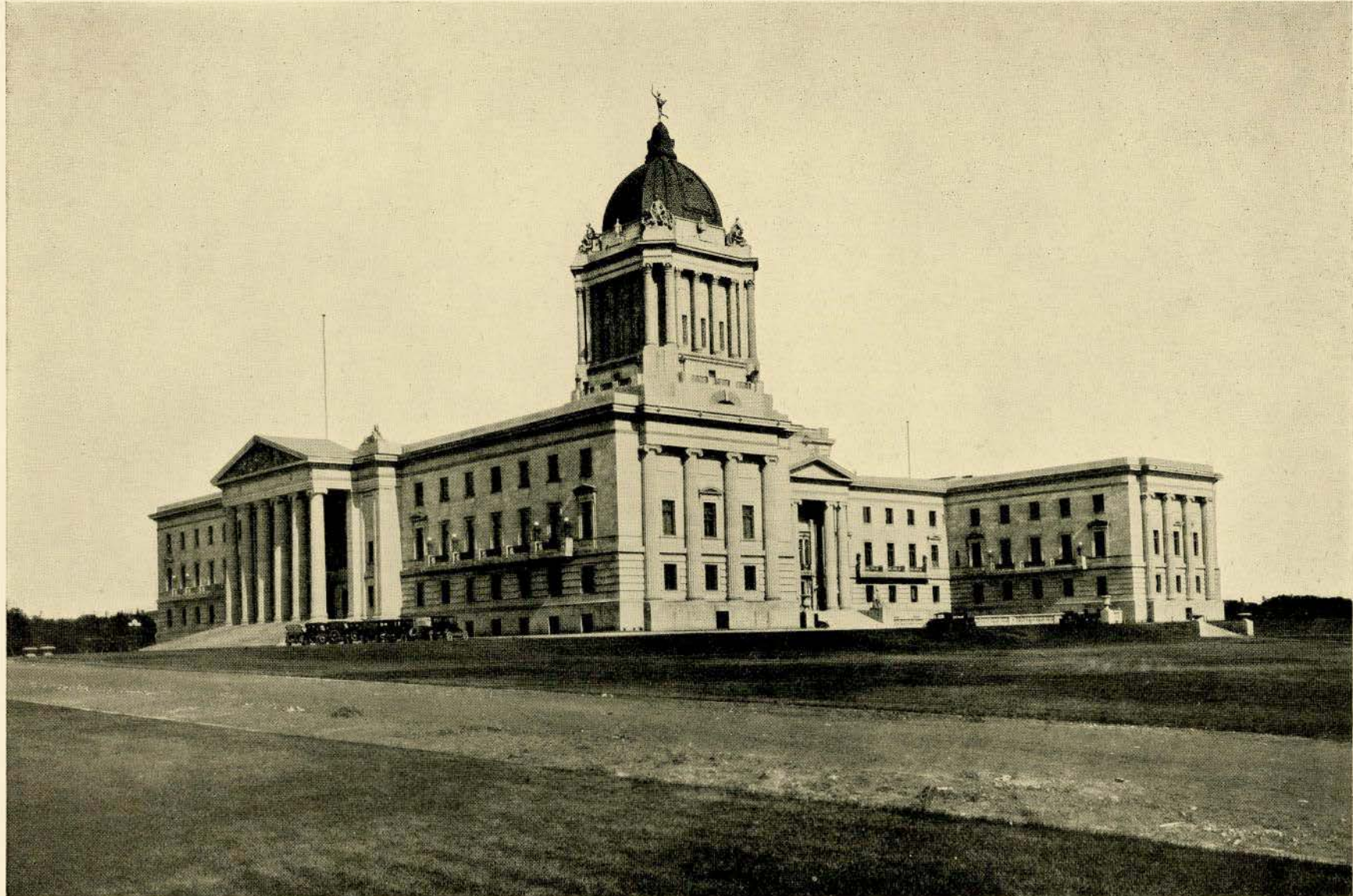
MANITOBA LEGISLATIVE BUILDINGS, WINNIPEG Frank W. Simon, F.R.I.B.A., Architect
