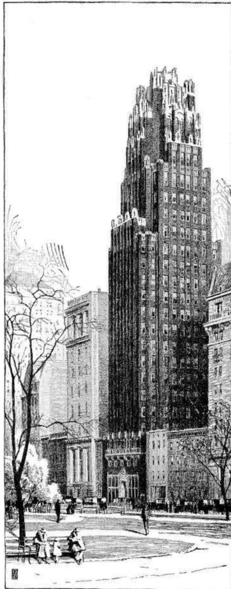
The American Radiator Company's new building is the only office building in New York City faced with black brick, with trimming in a rich golden color. Raymond Hood, Architect.
