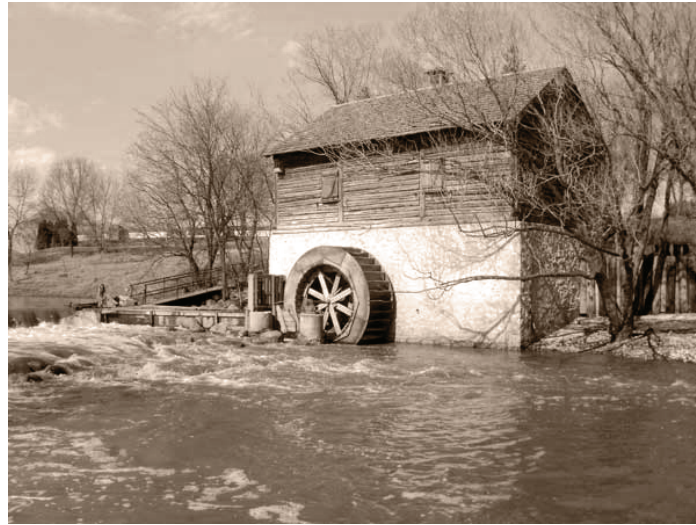
Figure 56. Grant's Old Mill, high river level. (Fraser 2011)
