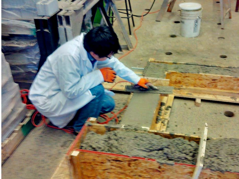
Figure 3.10 Concrete Surface Smoothing with Trowel
