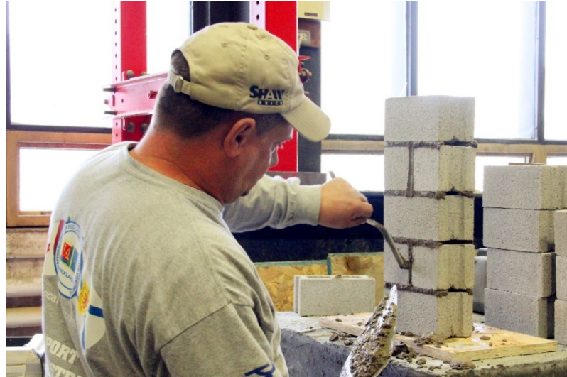
Figure 3.30 Construction of Masonry Prisms
