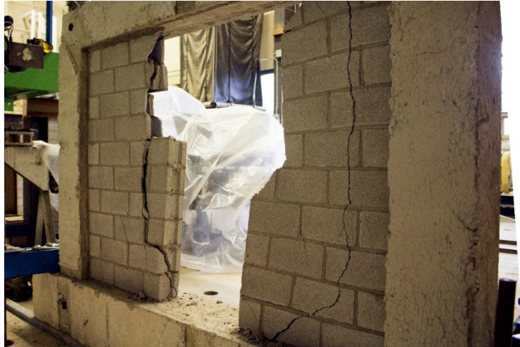
Figure 4.11 Failure Mode of Specimen IF-RC-DO on Windward
