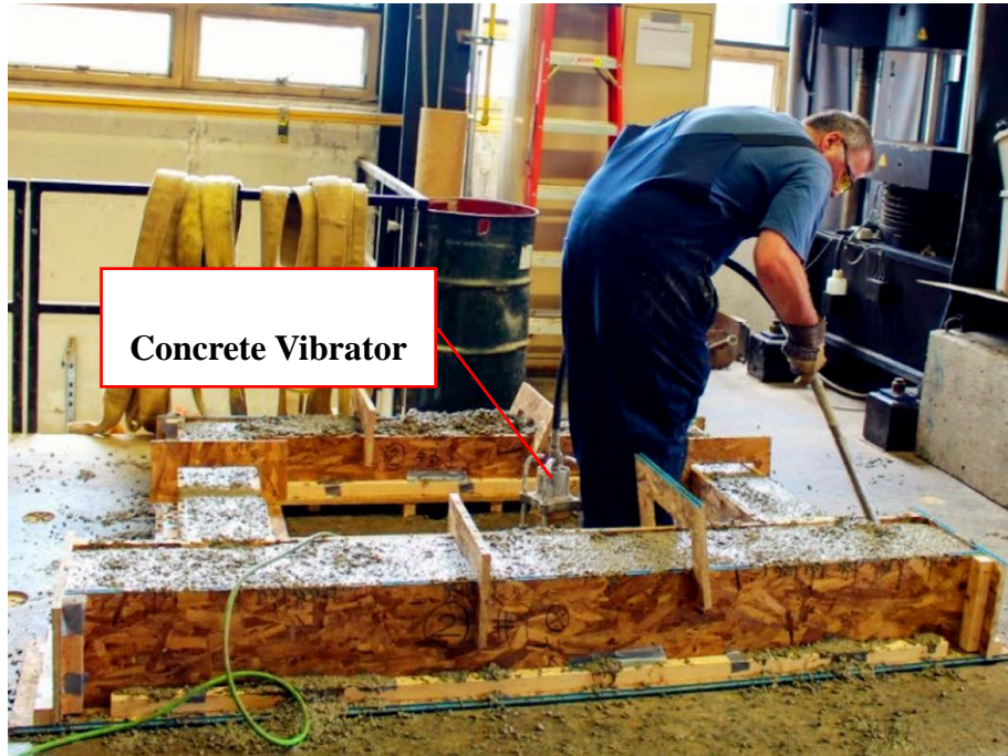
Figure 3.9 Concrete Casting and Vibrating
