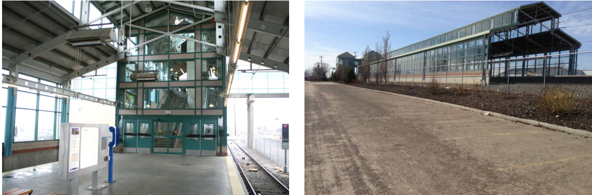
Images of the existing open air Belvedere LRT station structure showing the distinctive glass-walled shed form constructed from structural steel.
