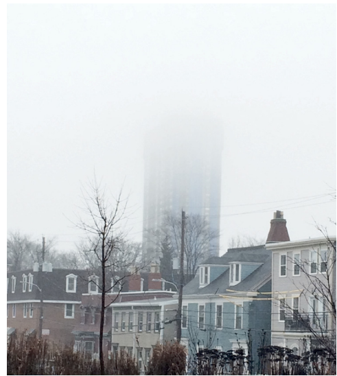
Figure 1: Fenwick Tower seen from Queen Street.
