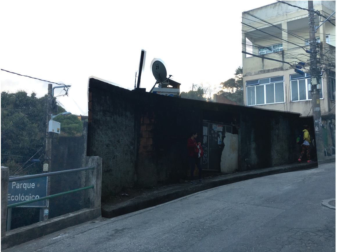
Image 50: Casa Deposito #1, Building site.
