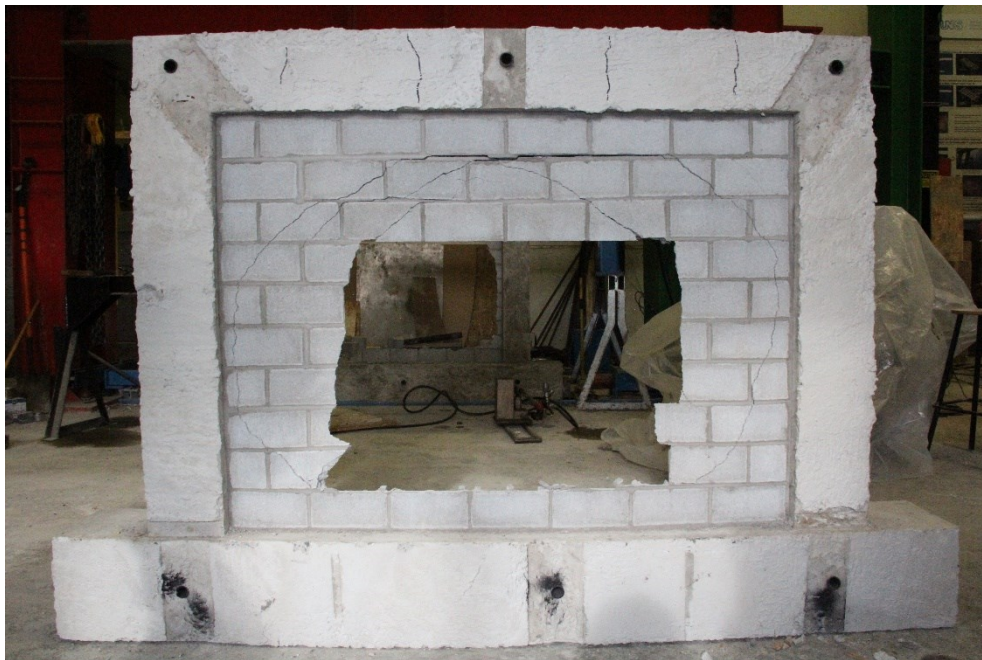
Figure 4.18 Failure Mode of Specimen IF-W-ND (Back View)
