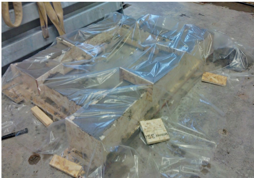
Figure 3.11 Curing of Concrete
