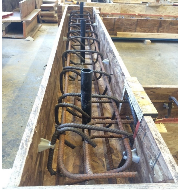
Figure 3.6 Formwork with Reinforcement, Chairs, and Tube Detail
