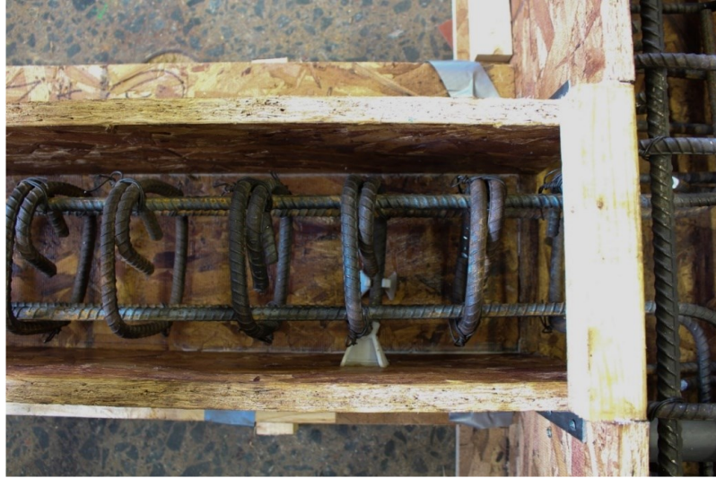
Figure 3.8 Details of Formwork with Reinforcement
