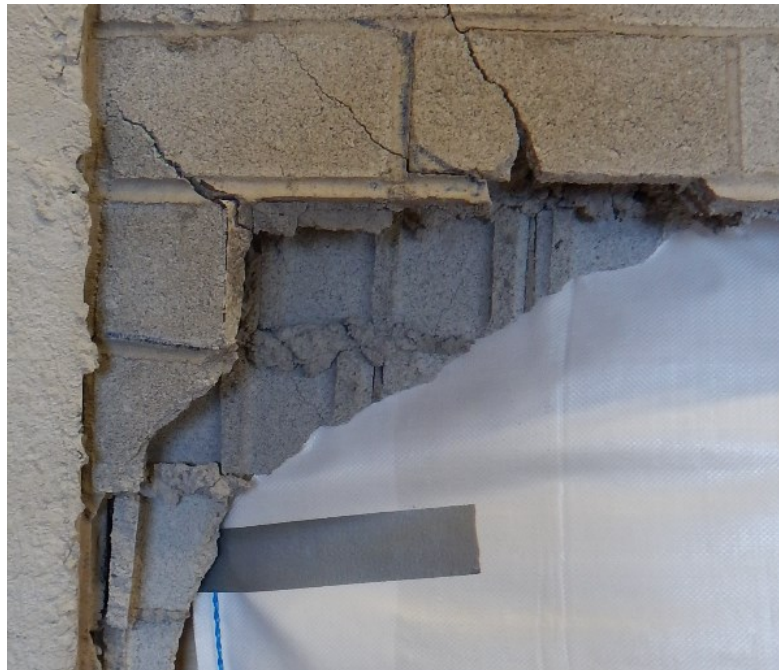
Figure 4.26 Web Shear Failure of Masonry Units for Specimen IF-D1
