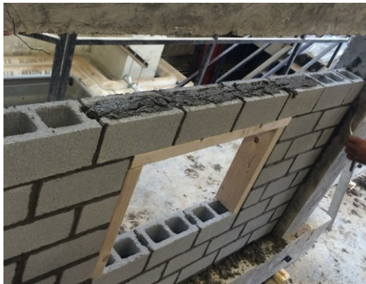
(e) Opening Construction Details
