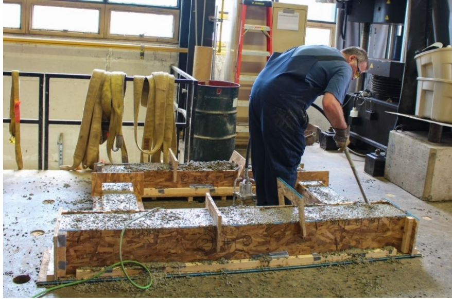
Figure 3.10 Concrete Pouring and Vibrating
