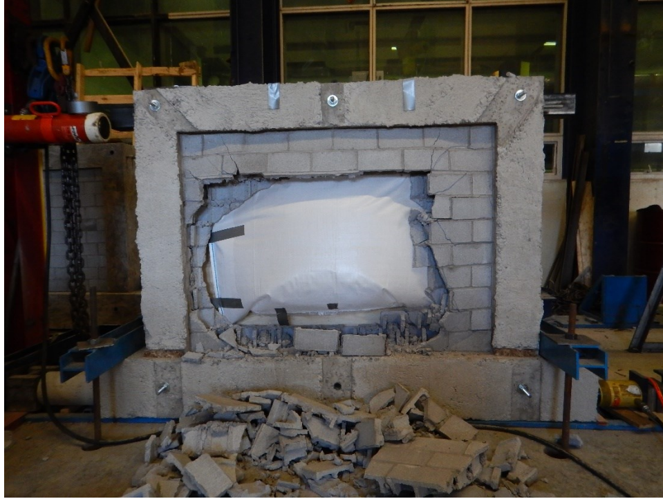
Figure 4.25 Failure Mode of Specimen IF-D1
