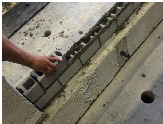
(c) Application of Mortar
