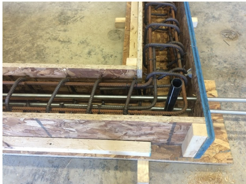
Figure 3.7 Formwork with Reinforcement, and Tube Detail
