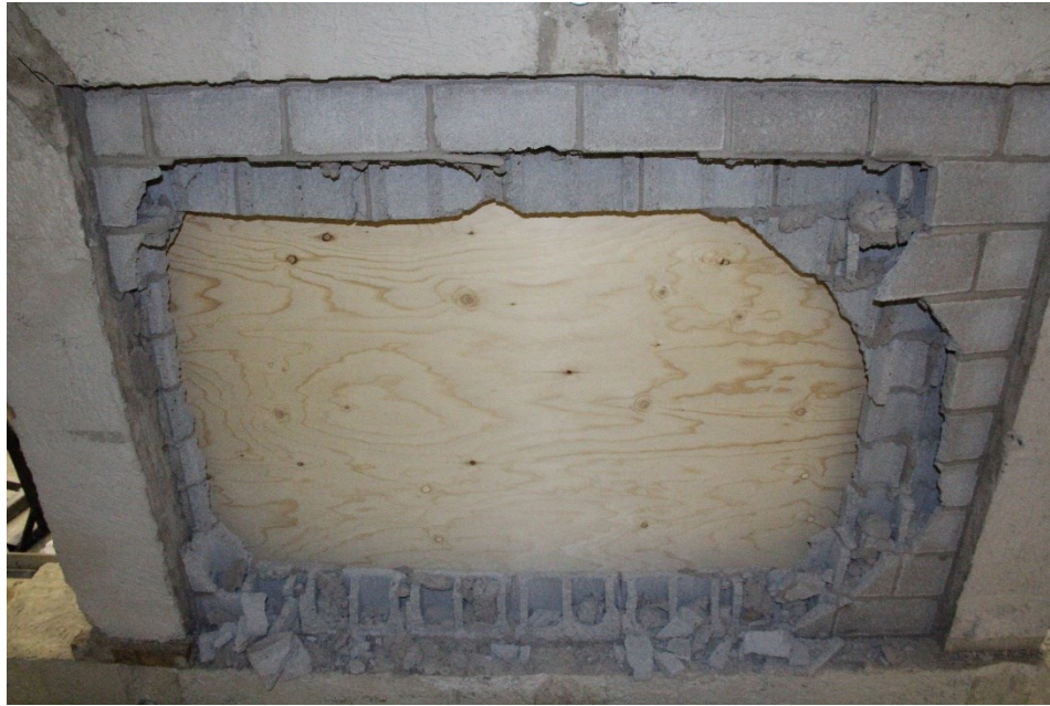
Figure 4.11 Failure Mode of Specimen IF-ND
