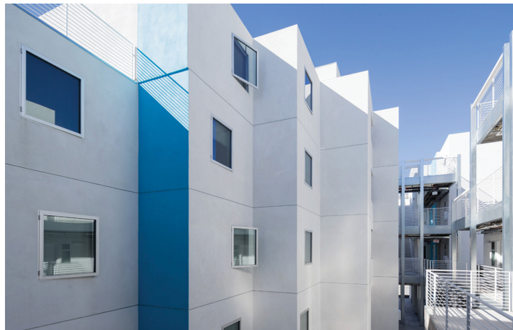
Figure 90: Photograph of interior courtyard/lightwell space of the third and fourth floor of Star Apartments. Photograph by Michael Maltzan Architecture 2016.
