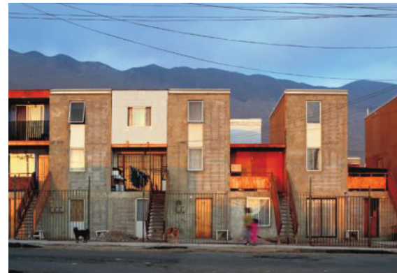
Figure 97: Photograph of a Quinta Monroy units, starting to be infilled by owners. Photograph by Elemental 2016.
