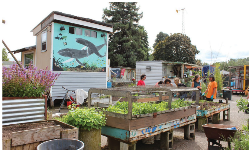
Figure 84: Photograph of the renovations done to a tiny house in Dignity Village. Photograph by Heben 2014.
