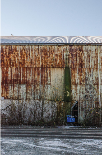
Figure 6: Photograph of Wilkinson Building being used as shelter by the unhoused
