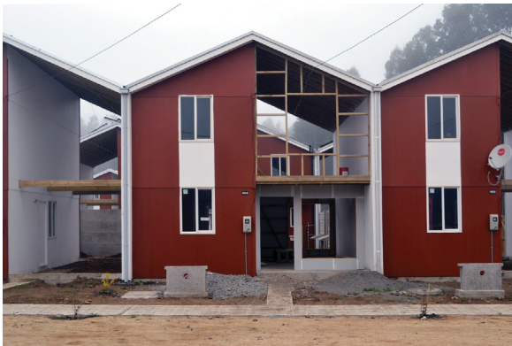
Figure 96: Photograph of a Villa Verde unit, starting to be infilled by owner. Photograph by Elemental 2016.
