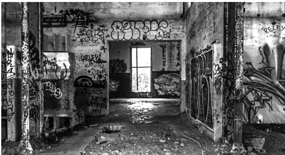
Abandoned Jordan River Generating Station; photograph by Darren Stone; from Vancouver Sun (2008).
