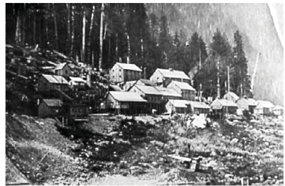
Tunnel Construction Camp 1903; Photograph from City of Vancouver Archives.
