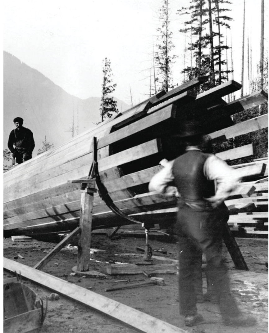
Wooden Penstock for Buntzen Lake Power Plant #1; photograph by Major James Matthews; from City of Vancouver Archives (1903).
