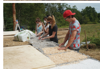
Tiny house . Deanery project freelab 2014. “Bagging” insulating materials within the floor joist cavities to reduce floor thickness.
