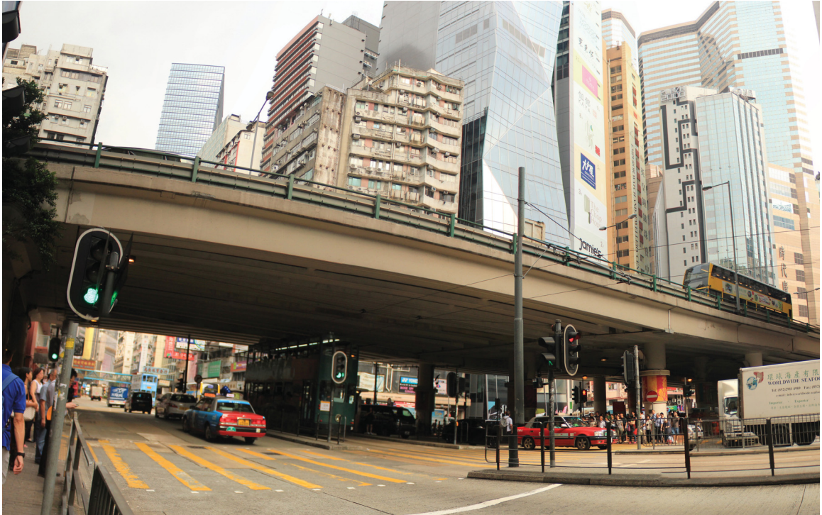
fig. 23.0. Typology II, a vehicular overpass in Causeway Bay. The intervention hopes to lift the user groups off from the sidewalk and away from the ground pollution.
