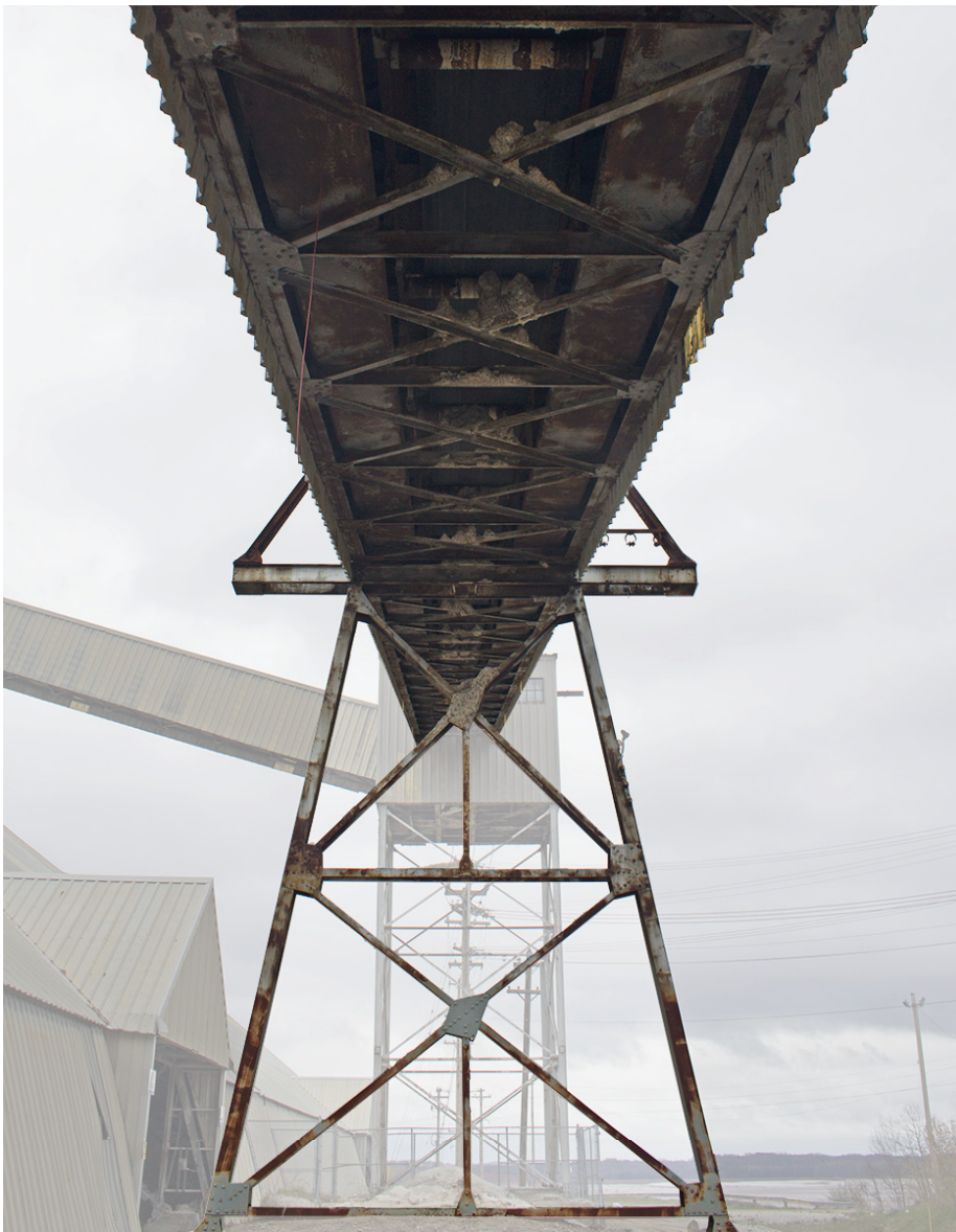
Site surroundings: Industrial infrastructure. Steel structure: cross-bracing, piers, and interior steel joists. Inspiration for the overarching structure of the creative hub.
