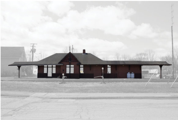
Vacant building: Civic.
