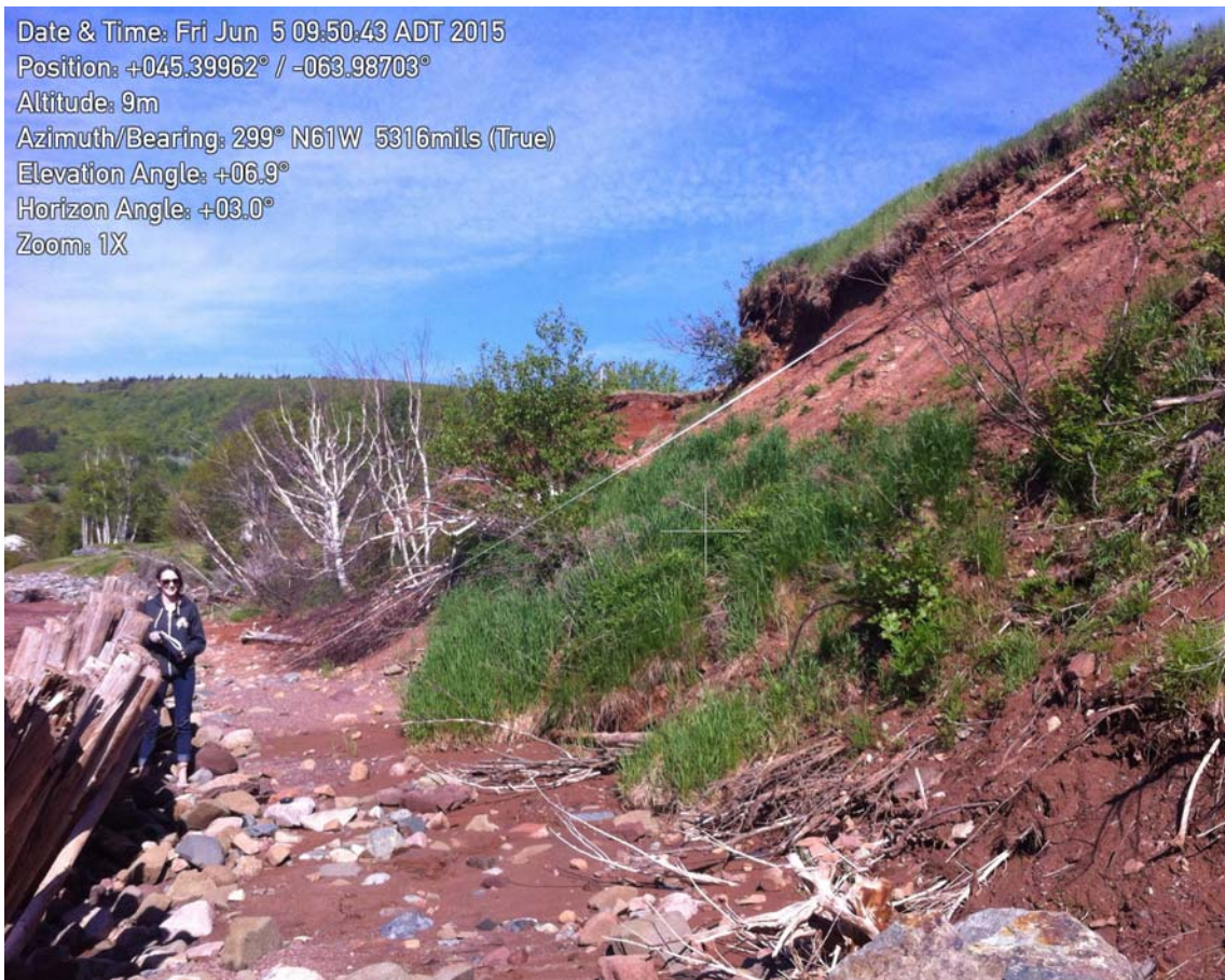
Figure 3.5: Erosion behind wall constructed against cliff base in 1987 in Lower Economy, Nova Scotia.
