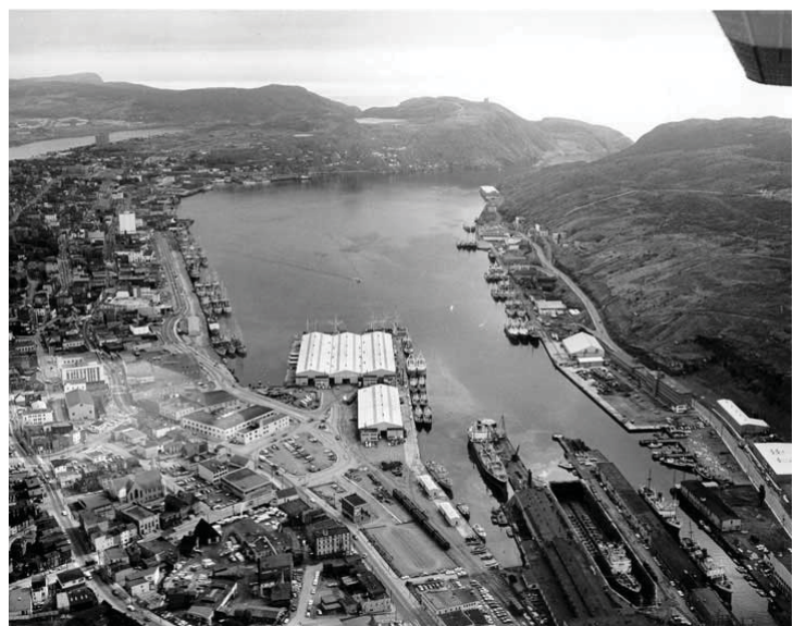
Complete harbour redevelopment (A Beautiful Sight 2015)
