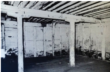
The Murray Premises rough post and beam construction contains knee bracing and joinery that reflect ship building techniques (St. John's Heritage Foundation 1977)
