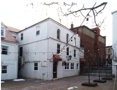
Murray Premises Courtyard, St. John's, 2015
