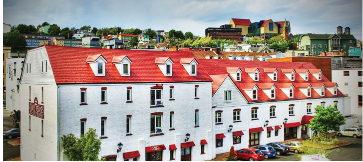
View of the renovated Murray Premises (Murray Premises Hotel 2014)
