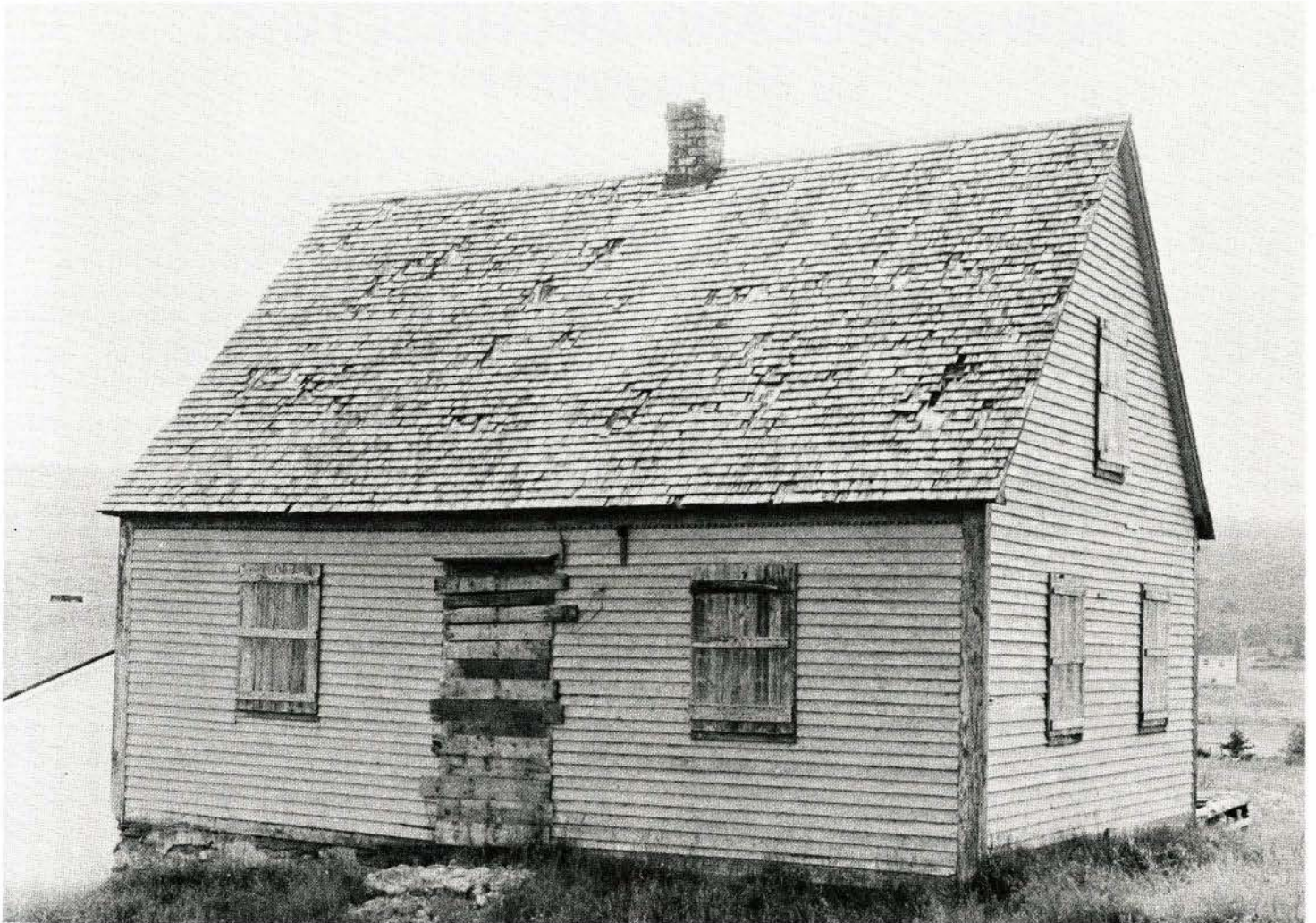
Plate 6 — Lundrigan house in Bay Bulls, Newfoundland. Typical one-and-a-half storey, central-hall plan with back kitchen.
