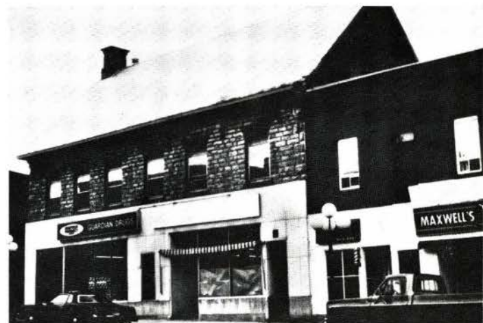
Local businesses often fail to maintain their buildings or have slip-covered them with layers of trendy materials.
