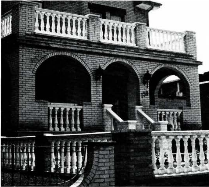
Facade renovation with balustrades and brick arches, Grace Street, Toronto.
