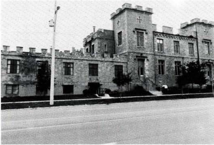
Wellington County Court House, North-East elevation—before.
