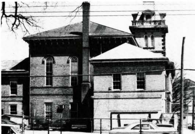
Simcoe Municipal Building, West elevation before.
