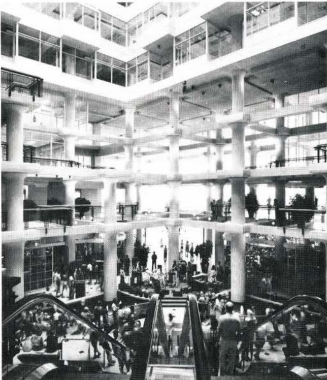
South atrium looking towards the south-east harbour. Note mushroom capped columns.
