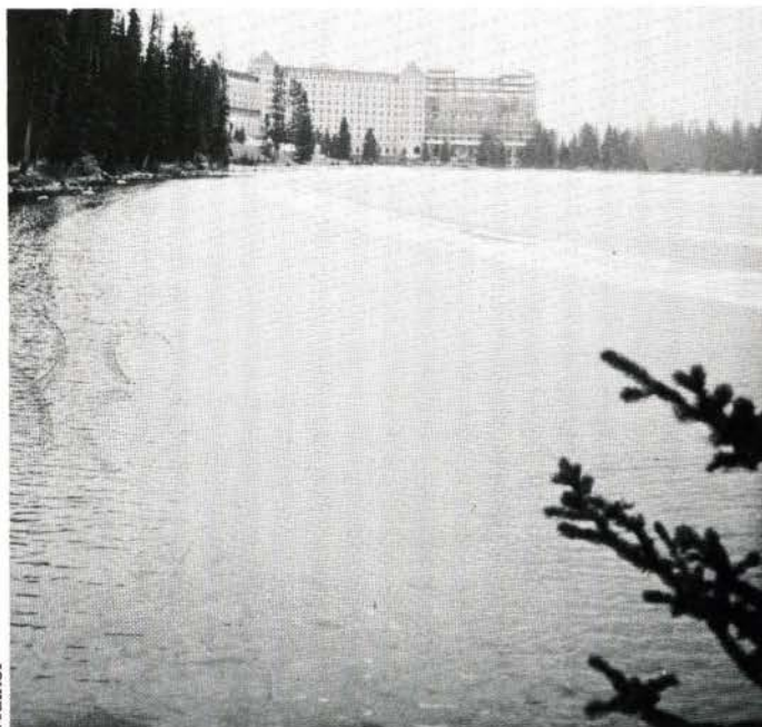
Figure 18. Chateau Lake Louise with new wing under construction, 1987.
