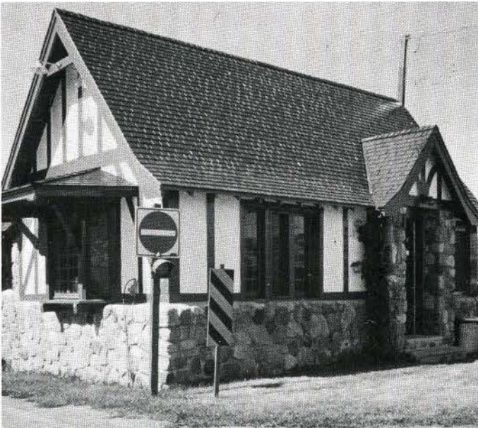
Figure 9. Registration building, Waterton National Park.
