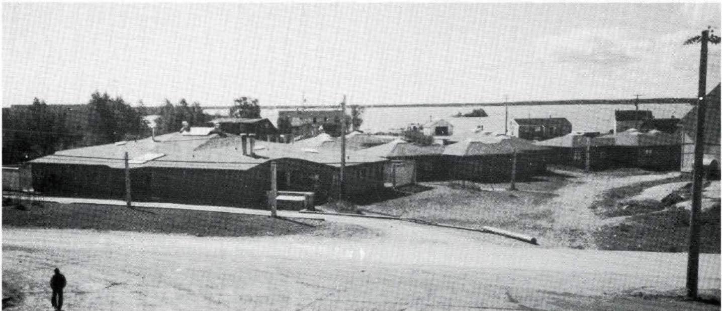
Seniors Home in Rae NWT. The design is composed of cabin-like units to relate to the traditional lifestyle of the elders in the community.
