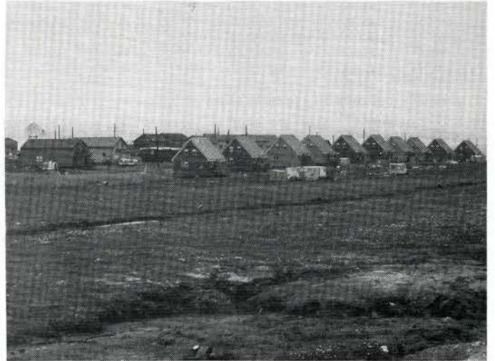
Pond Inlet, N.W.T. - rows of houses.
