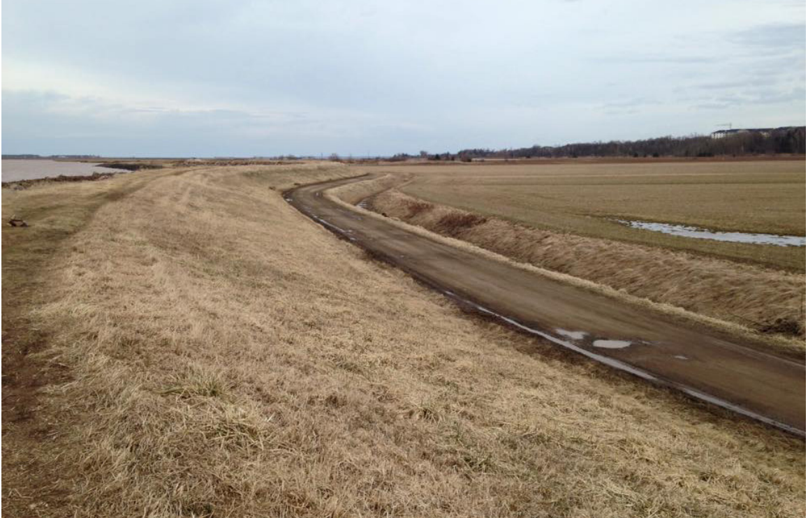
Pathways exist on top of and adjacent to existing dike seen here in eastern Wolfville. The Minas Basin can be seen on the left at mid/high tide, and farm land can be seen on the right with a drainage channel (polder) running in between pathway and field.
