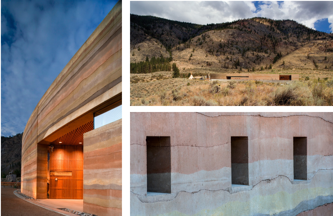
Nk'Mip Desert Cultural Center, Osoyoos, BC, Canada. HBBH Architects. Left: Night time image of the rammed earth exterior wall, Top right: The architecture completely blends in to the landscape, Bottom right: Window detail in rammed earth wall.
