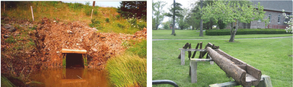
Left: Existing aboiteau in an Annapolis Valley diked farm land, Right: A recovered aboiteau, circa 1700s, discovered at Grand Pré.
