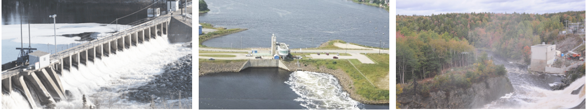
Damage to the surrounding natural environment is seen in images of these three examples of Nova Scotia dams. From left to right: Malay Falls, Annapolis Royal Tidal Dam and Sissiboo Falls
