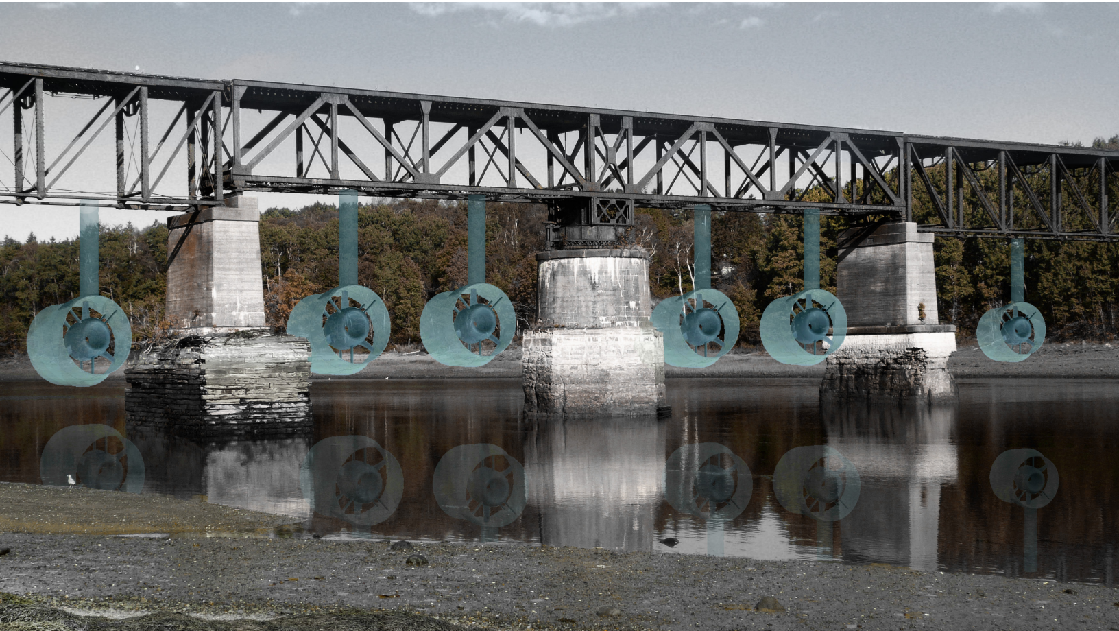
Small scale tidal turbines installed under the Avon River rail bridge at low tide.
