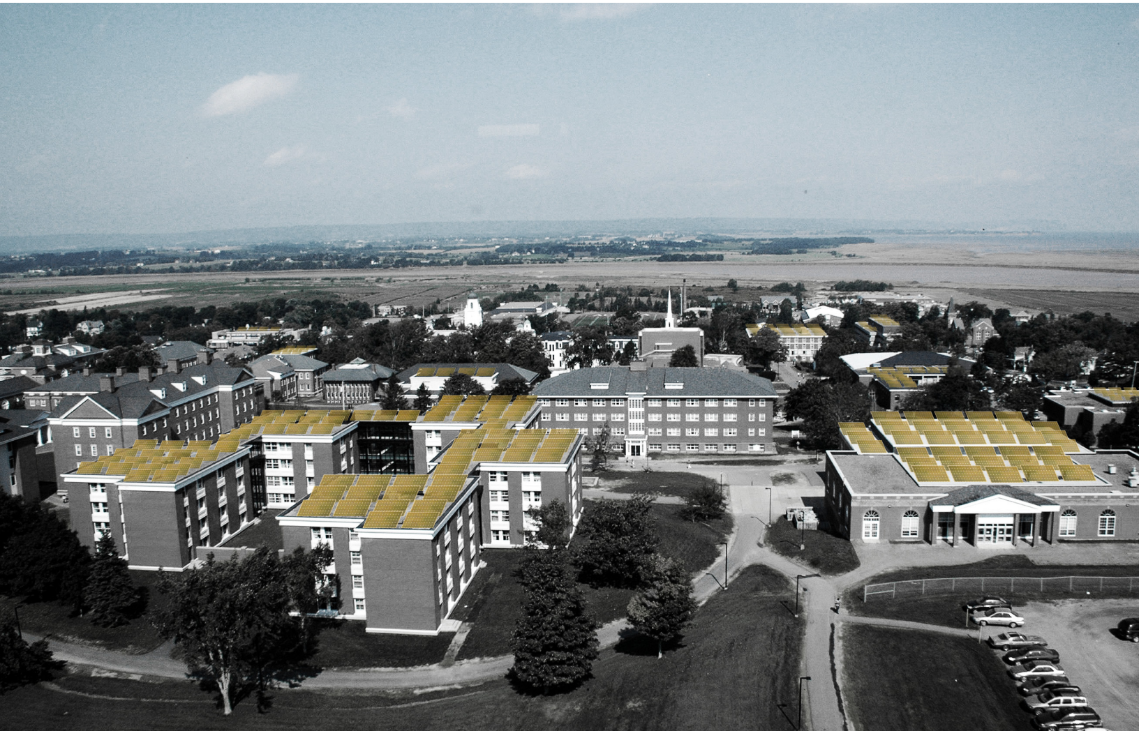
Solar panels installed on Acadia University rooftops.
