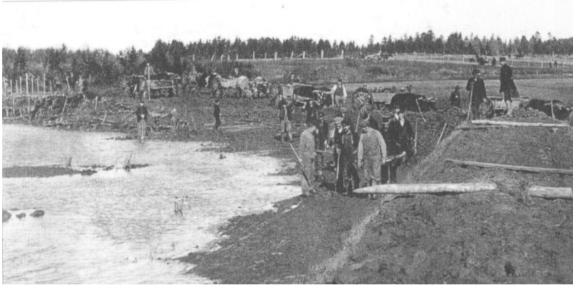
An image showing the collaborative nature of dike building and maintenance. This image was taken by A.L. Hardy in 1913 and shows men repairing the Davidson Aboiteau and dike wall on Long Island, Grand Pré; from Bleakney, Sods, Soils & Spades , 39.
