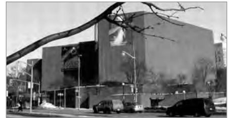
FIG. 8. VIEW OF THE NAC FROM THE SOUTHWEST ALONG ELGIN STREET. | RHONA GOODSPEED, PARKS CANADA, 2005.
