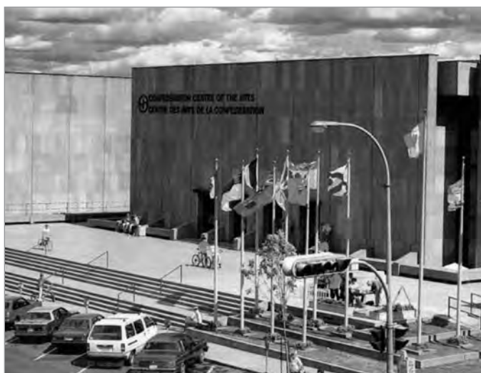
FIG. 34. CONFEDERATION CENTRE OF THE ARTS, CHARLOTTETOWN, PRINCE EDWARD ISLAND; BUILT IN 1964; AFFLECK, DESBARATS, DIMAKOPOULOS, LEBENSOLD, SISE, ARCHITECT. MAIN ELEVATION ABOVE, TERRACE ON LOWER RIGHT, AND INTERIOR VIEWS FROM MEMORIAL ON LOWER LEFT. | REPRODUCED FROM GENEVIÈVE CHARROIS, "LE CENTRE DES ARTS DE LA CONFÉDÉRATION," HSMBC, SUBMISSION REPORT 2002-45.
