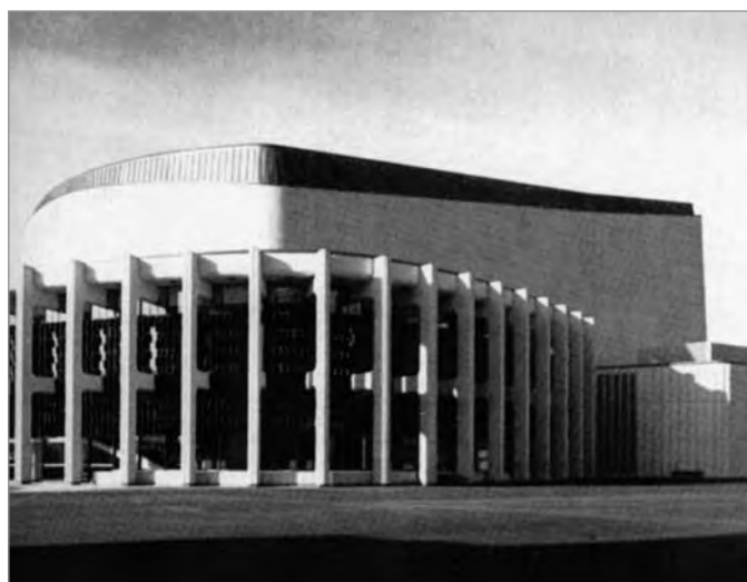
FIG. 35. PLACE DES ARTS, MONTRÉAL, QUÉBEC, SALLE WILFRID-PELLETIER; BUILT IN 1963, AFFLECK, DESBARATS, DIMAKOPOULOS, LEBENSOLD, MICHAUD, SISE, ARCHITECT. | JOURNAL OF THE ROYAL ARCHITECTURAL INSTITUTE OF CANADA (JRAIC) , NOVEMBER 1964, P. 123.
