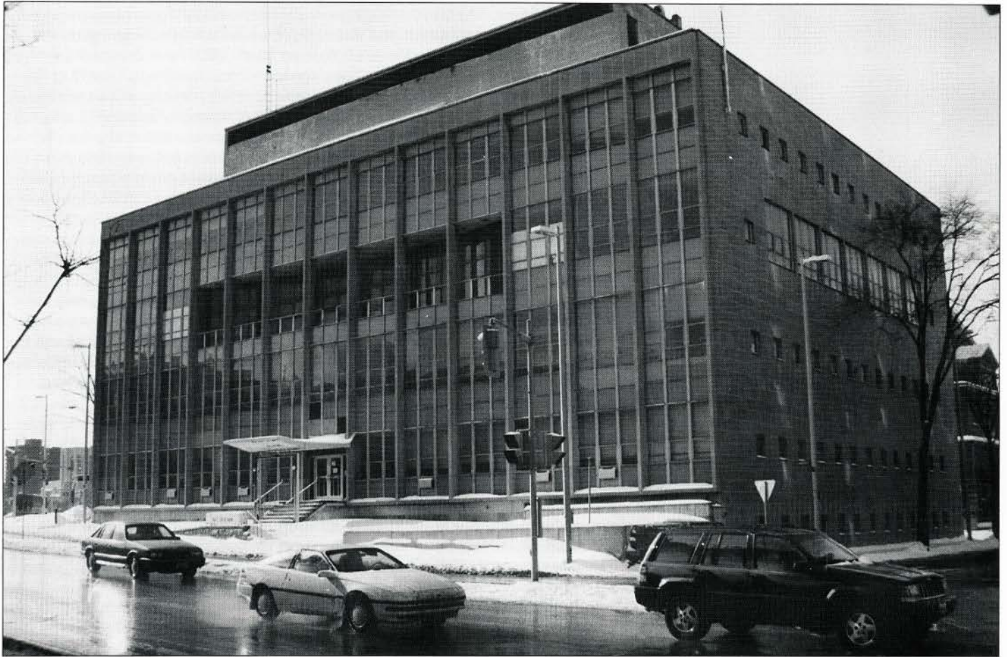
Figure 1. The former Police Station, 60 Waller Street, Ottawa, Peter Dickinson, architect, 1954-57; demolished in 1994. (Dan Grant, Image [Sandy Hill], 1994)
