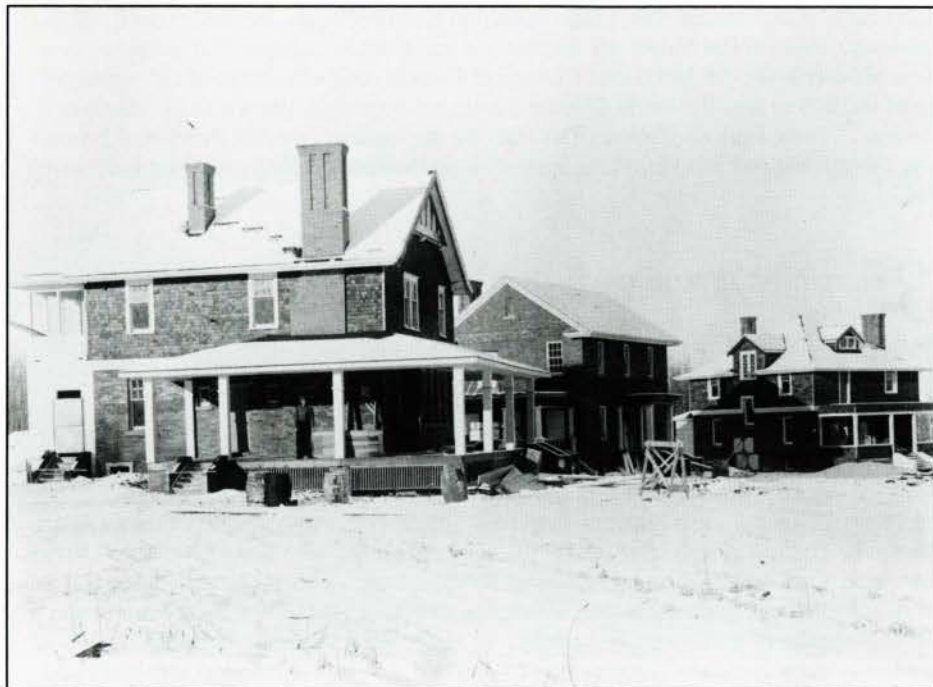
Figure 5. Professors' houses under construction at the University of Alberta, 1912; view from the southeast. (University of Alberta Archives, accession no. 69-12-242)
